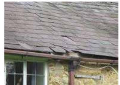
Damaged and slipped slate tiles
