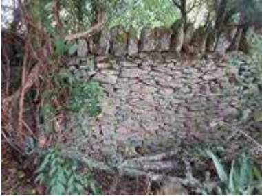
Existing dry stone boundary wall ( to left of site )
