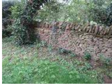
Existing dry stone boundary wall ( to the right of site )
