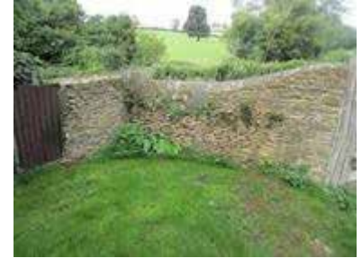
Existing dry stone boundary wall ( to the right of site )
