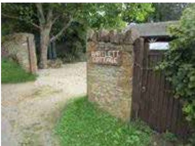
Existing pedestrian gate and missing vehicle gate
