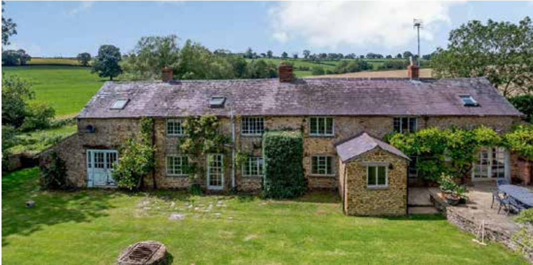
Views of the existing south-east (garden) elevation
