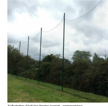
A) Illustration of ball stop fencing example - permanent type.
