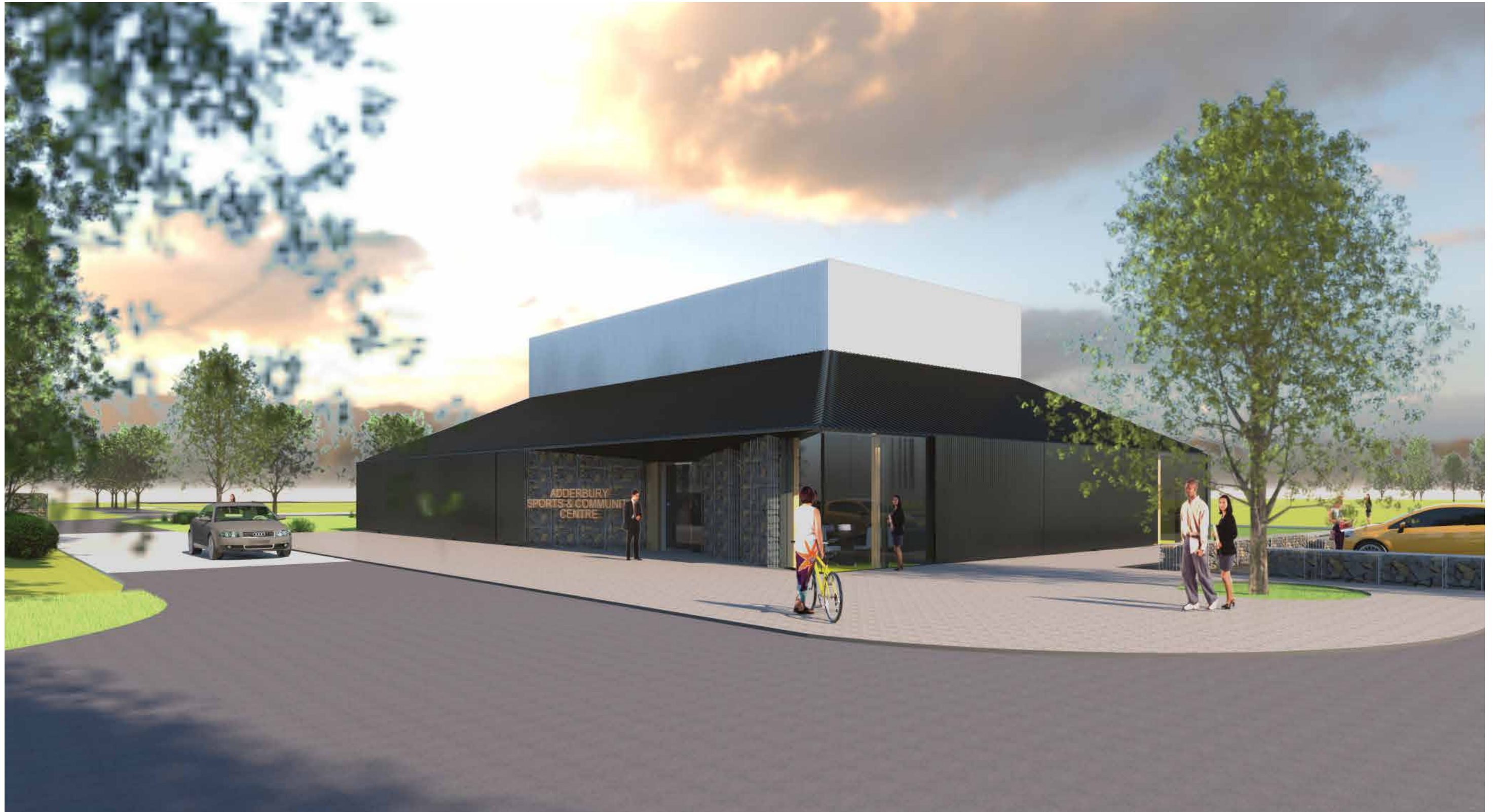
Fig 42: View from Milton Road showing local hornton stone in gabion baskets, used to frame entrance to new building
