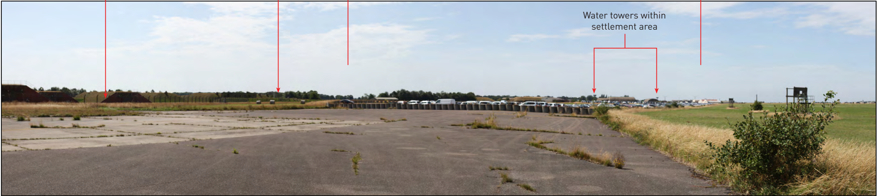
On the southern taxiway next to the proposed car storage area
