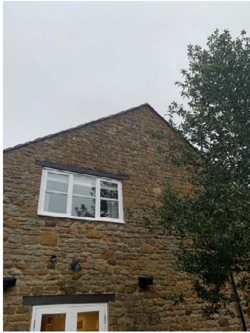
Western Gable elevation showing good condition of the stonework.
