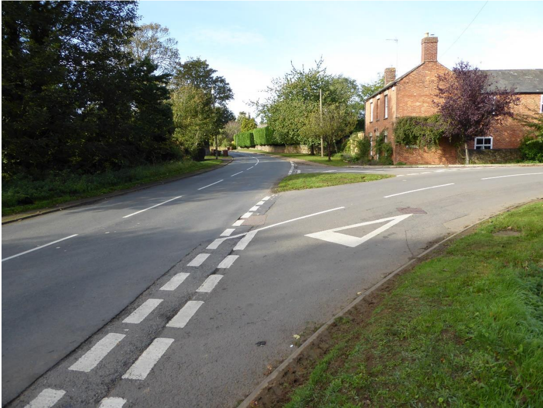
1. View of 'blind' bend looking west from junction of Clifton Road with Earl's Lane
