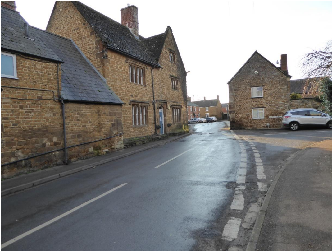
1. B4031 main west-east route pinch-point between Castle Street and Chapel Square looking west towards village centre. Note the lack of footways on either side.
