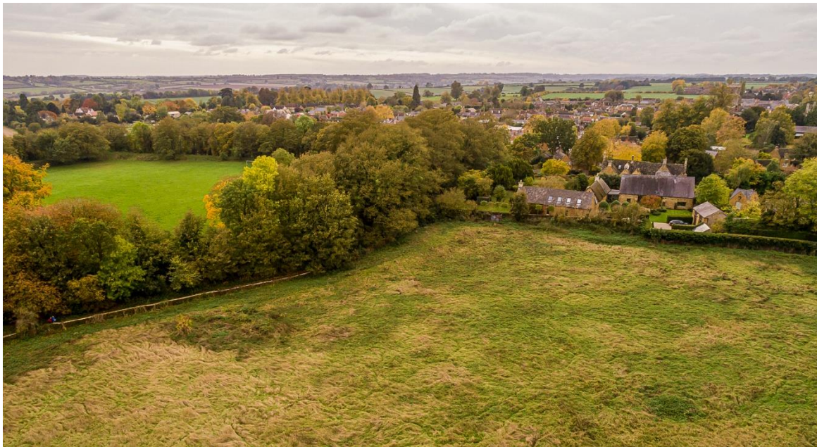
2. Aerial view of The Poplars in autumn looking west towards the Castle Bams on its western boundary, with Castle End behind. The open green space surrounded by trees in the top left is the interior of the western part of the western bailey.
