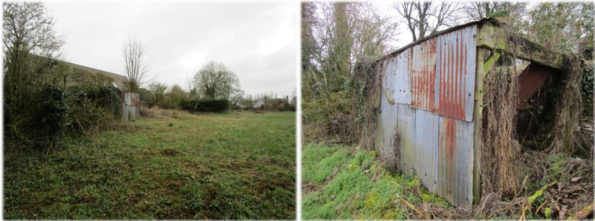
Western boundary stone wall with scrub (left) and dilapidated tin shed (right)
