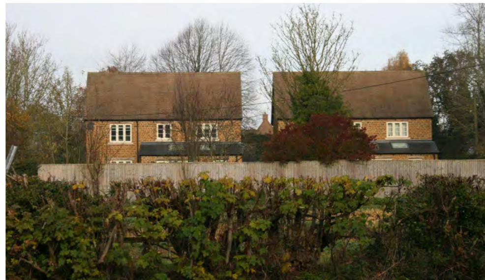
Existing modern ironstone houses to north of site
