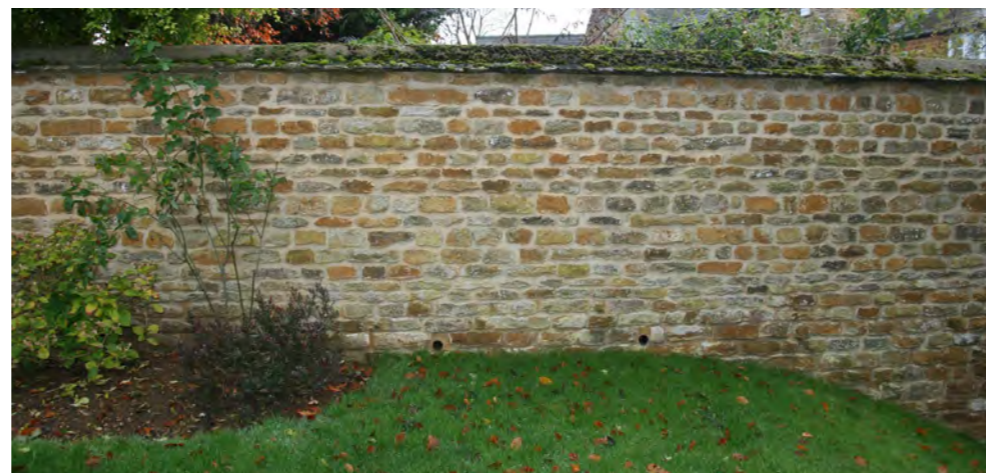
Existing stone wall running along Castle Street
