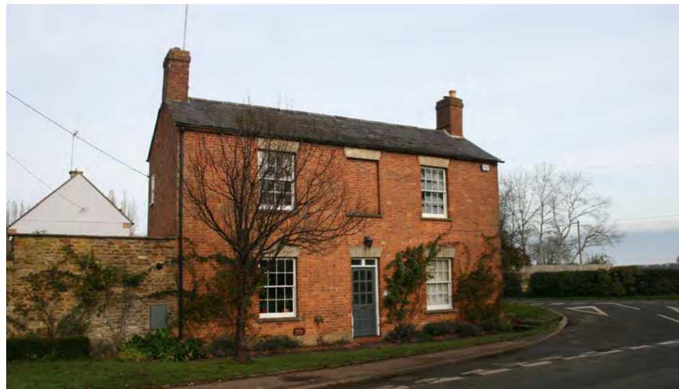
Existing brick house to north west
