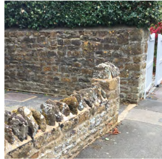
Timber 5-bar gates and stone-on-edge coping are common within the context
