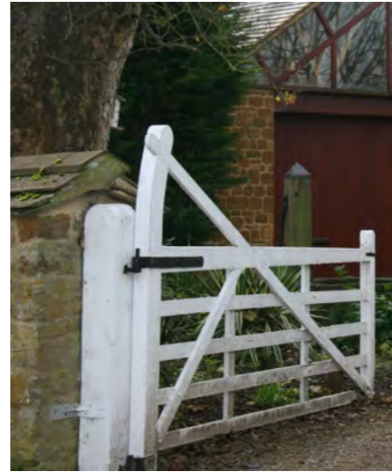
Timber 5-bar gates and stone-on-edge coping are common within the context
