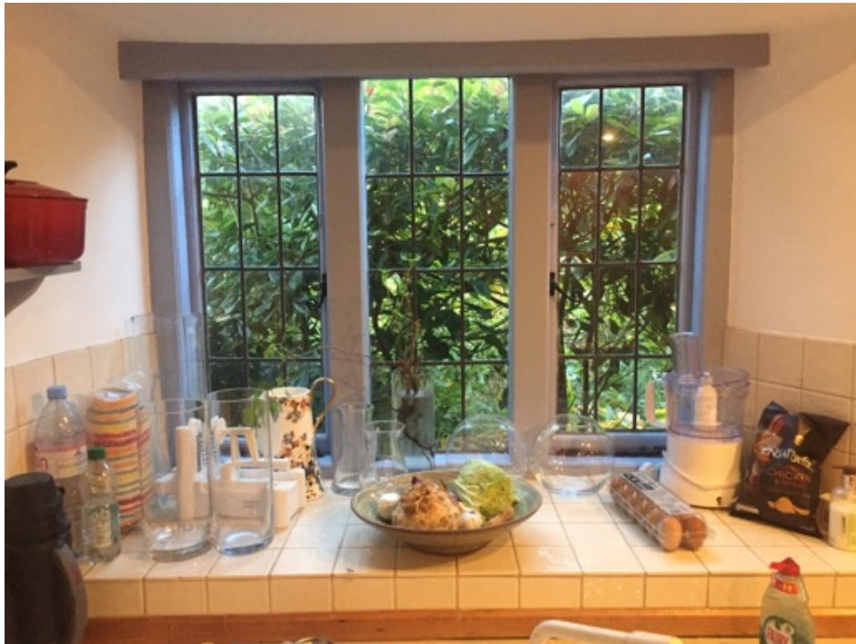
Detail of the window with modern fixed and opening timber casements
