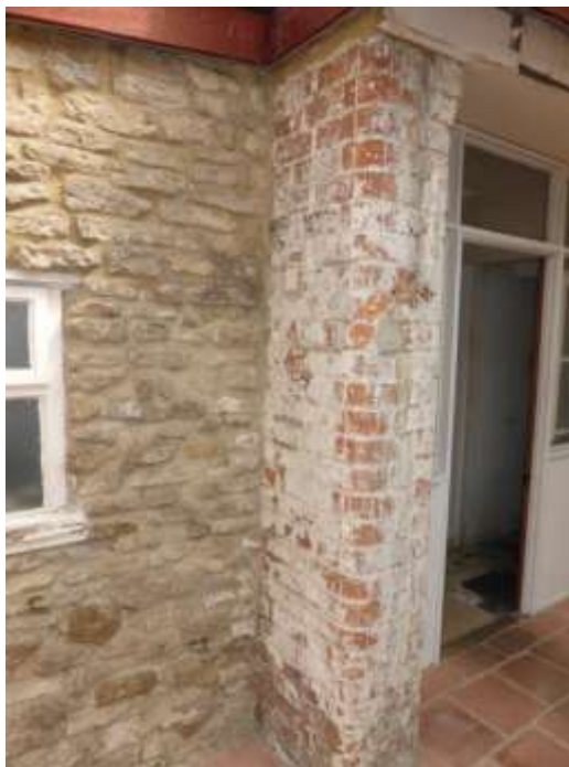
Figure 33: Brick pier at the western end of G7
