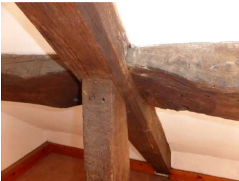
Figure 56: Tenoned purlin in A1
