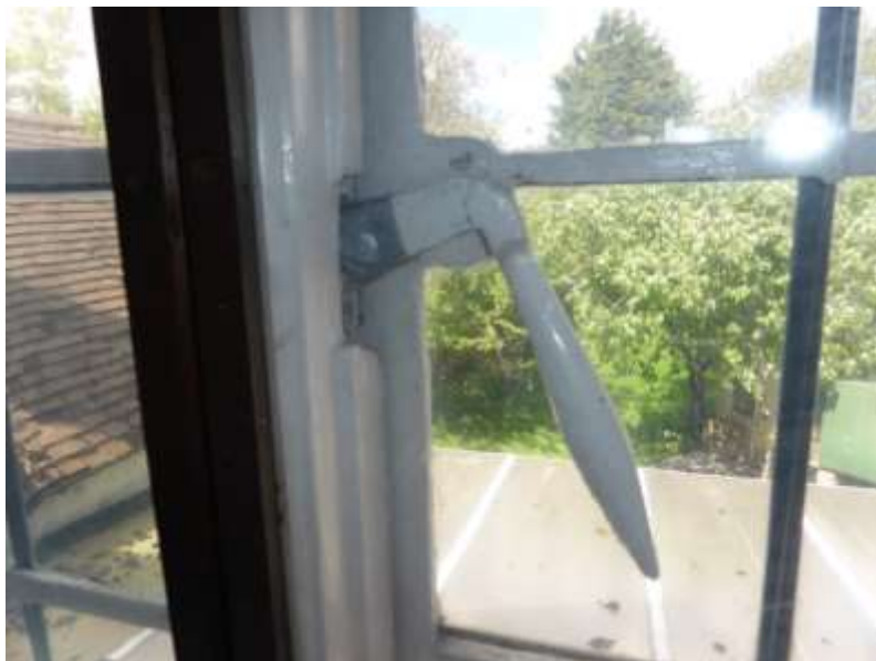
Figure 46: L-shaped bar catch to the central casement of the thermal window in F3
