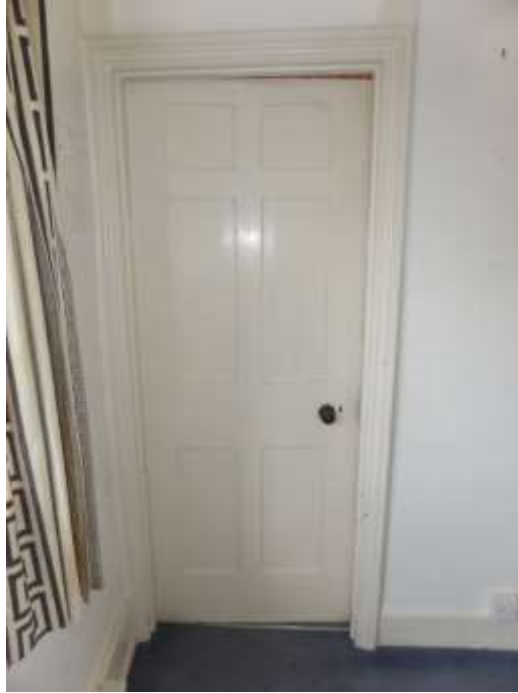
Figure 45: Early 20 th century door to F3
