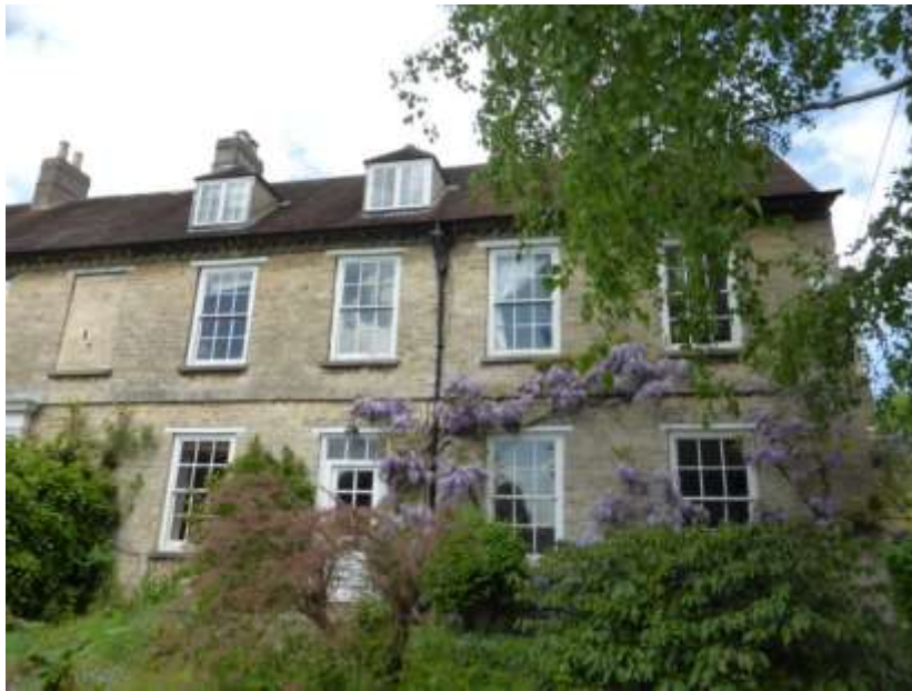
Figure 4: Front elevation of Wendlebury Lodge
