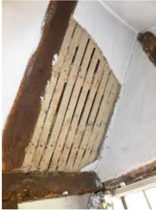
Figure 61: Rear dormer in A5 with sawn laths and plaster finish
