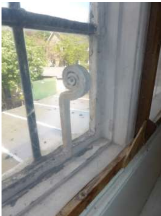
Figure 43: Detail of the spiral casement handle of the thermal window
