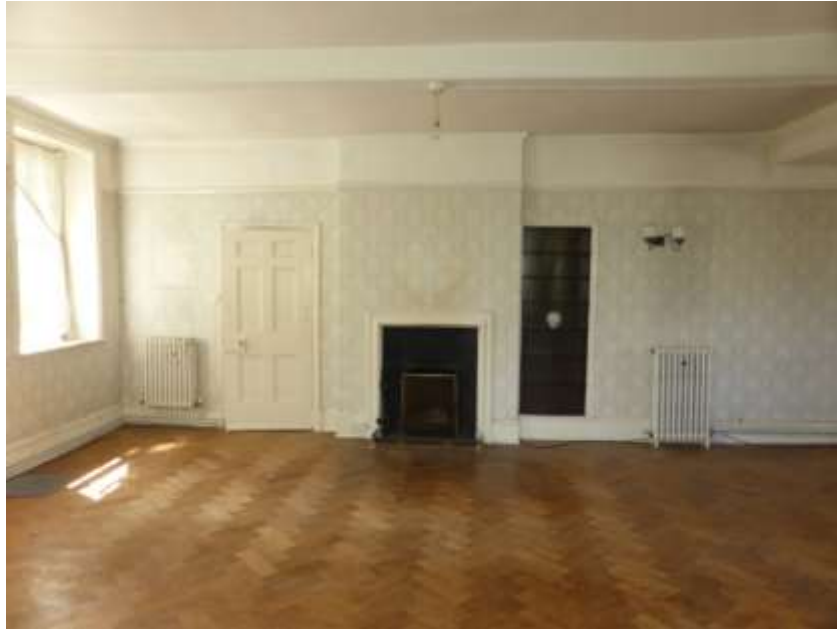
Figure 48: West wall of Bedroom F5
