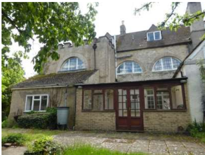
Figure 13: Rear elevation of Wendlebury Lodge
