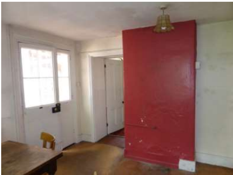
Figure 36: Early 20 th century chimney breast along the south wall of G10
