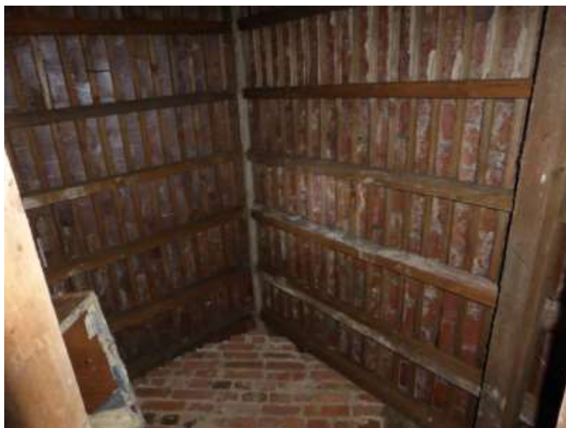
Figure 37: Common rafter roof over G10
