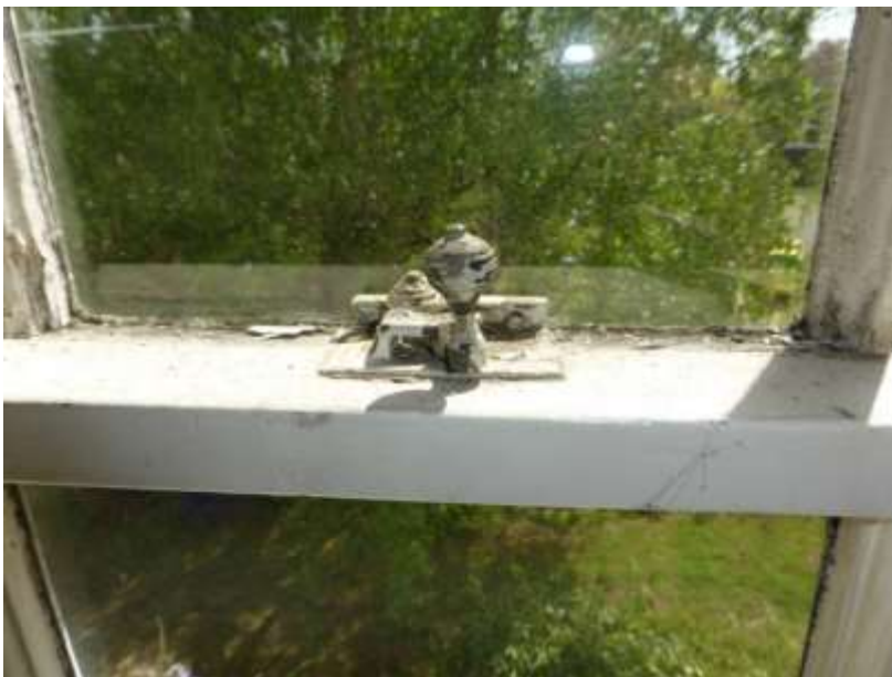
Figure 51: Later 19 th century type sash fasteners in F5
