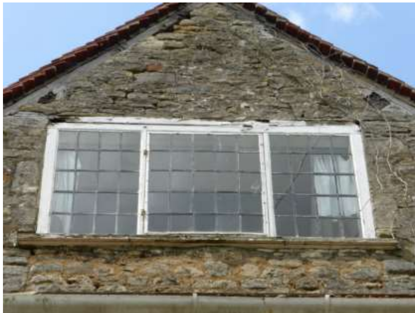
Figure 11: Late 19 th to early 20 th century metal casements to the attic
