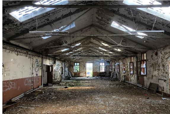
10. Interior of building in 2019
