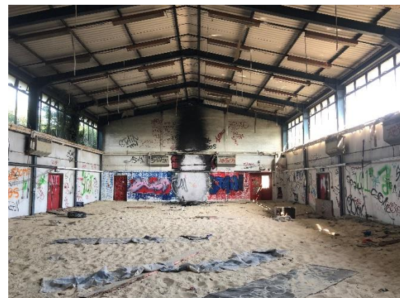
6. Interior of Building 886
