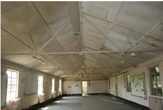
9. Interior of building in 2013
