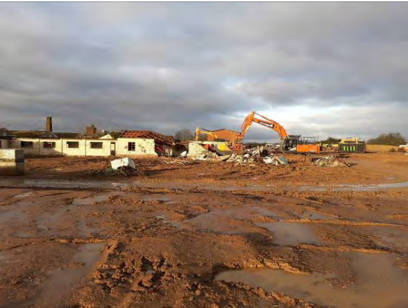
02.02.21 – Building demolition in north
