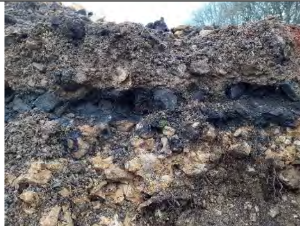
28.04.21 – Black gravel present below surface cover of reworked natural (0-0.2m) and underlain by natural limestone gravel
