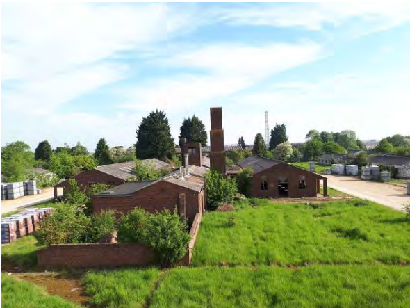
22.05.18 – Former boiler house in the centre of the site (chimney) with USTs
