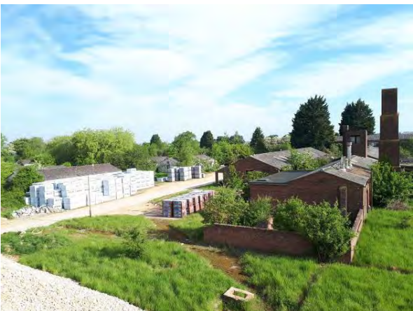
22.05.18 – Northwestern view across site
