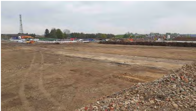
13.05.21 – North-eastern view following completion of works
