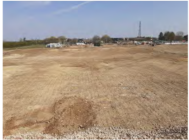
20.04.21 – Northern view across site
