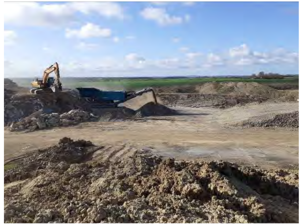
06.04.21 – Crushing site-won hardstanding commencing
