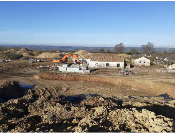
09.03.21 – Western view across the southern half of the site
