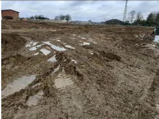
17.02.21 – Location of Hydrock hotspot located by GPS
