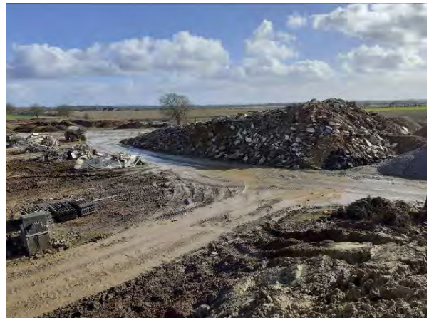
16.02.21 – Stockpile of recovered hardstanding prior to processing
