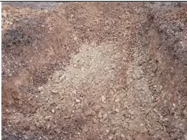
17.02.21 – Excavation of second trench to 1.1m bgl
