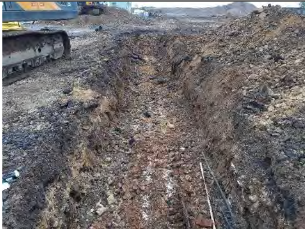
28.04.21 – Excavation of trench 1 within Hydrock hotspot area TP102.
