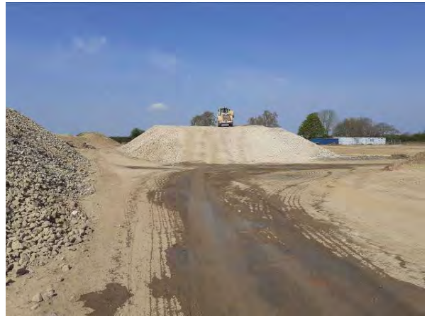
20.04.21 – Dust suppression taking place during dry conditions
