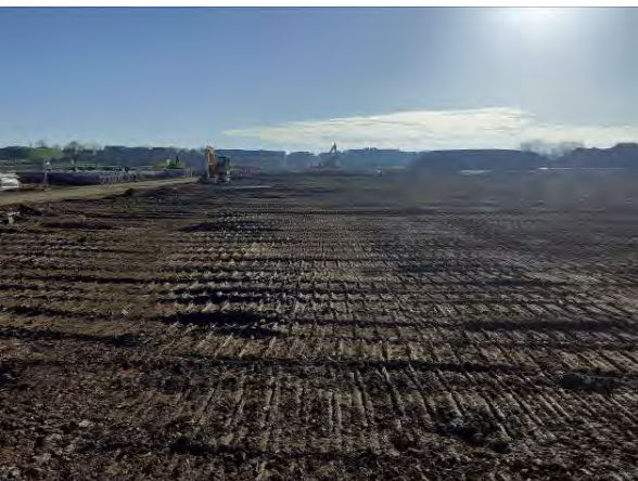
09.03.21 – Eastern view following regrade completion
