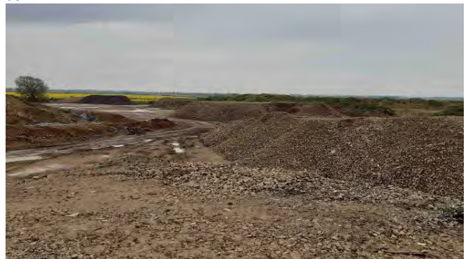
13.05.21 – Stockpiles of site-generated aggregate present in the south
