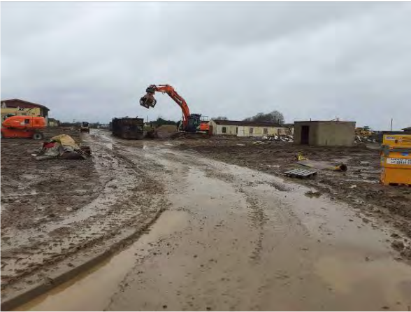
20.01.21 - Recovery and recycling of demolition materials
