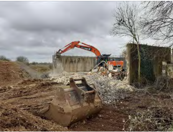
16.02.21 – Breaking out of walls around former substation
