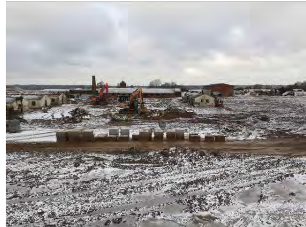
08.02.21 – Regrading to east of boiler house
