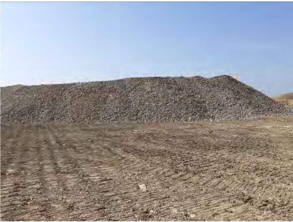
20.04.21 – Stockpile of site-generated aggregate (Agg-SP2)
