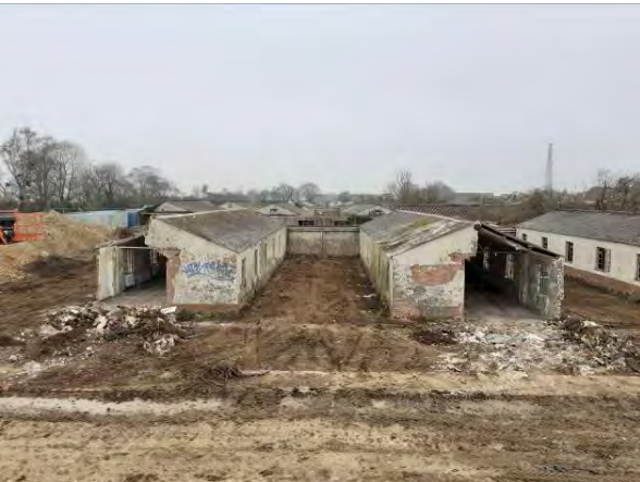
02.03.21 – Northern view of site from southern end. Buildings awaiting ACM strip
