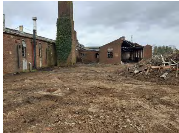
16.02.21 – Turf recovery of verge area around boiler house
