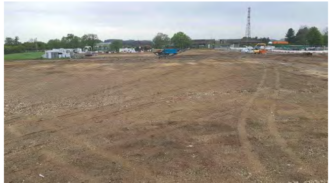
13.05.21 – Northern view following completion of works
