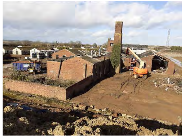
16.02.21 – ACM strip from boiler house
