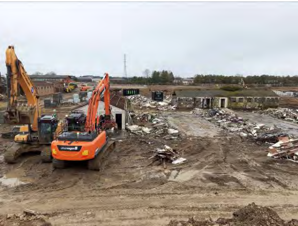
16.02.21 – Building demolition in south
