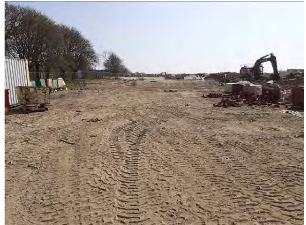
20.04.21 – Eastern view across the north of the site
