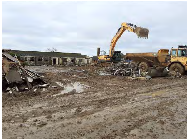
02.02.21 – Recovery of metal and wood wastes following building demolition for recycling
