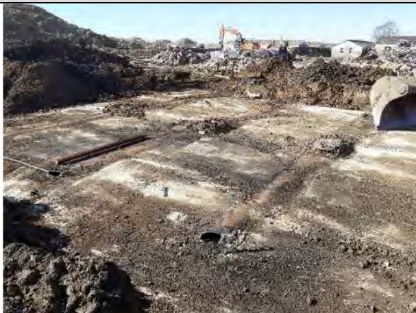
09.03.21 – Exposure of tank locations following demolition of boiler house
