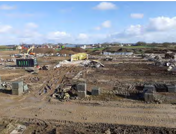
16.02.21 – Eastern view across site within area of recent building demolition
