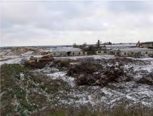
08.02.21 – Western view across site from eastern boundary
