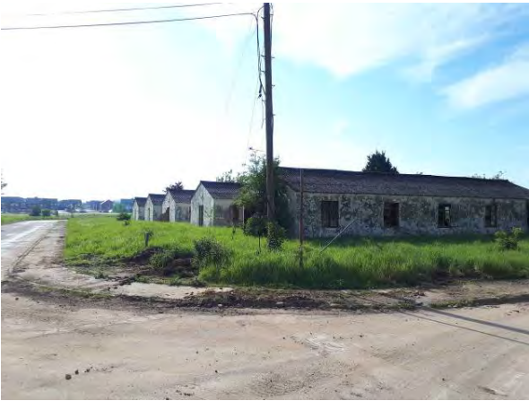
22.05.18 – Eastern view across north of site. Derelict buildings lined across site associated with former school classrooms.
