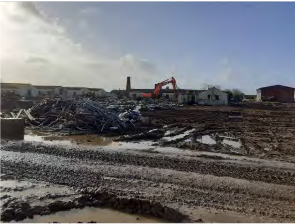
02.02.21 – Building demolition and hardstanding removal
