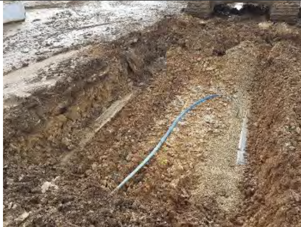
17.02.21 – Excavation of trench to 0.8m due to presence of possible drain and water pipe
