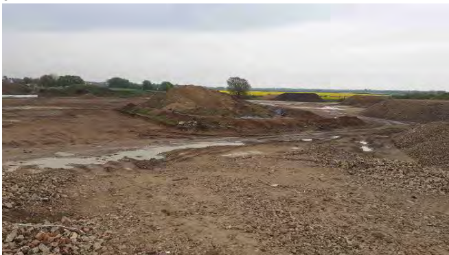
13.05.21 -South-eastern view. Temporary stockpile of contaminated soils from Phase 9 baseball pitch remains within quarantine area
