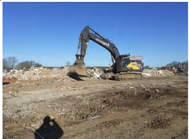
09.03.21 – Breaking out of hardstanding (slab) below demolished building footprint
