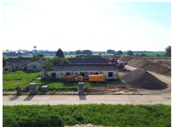
22.05.18 – Eastern view across the southern half of the site
