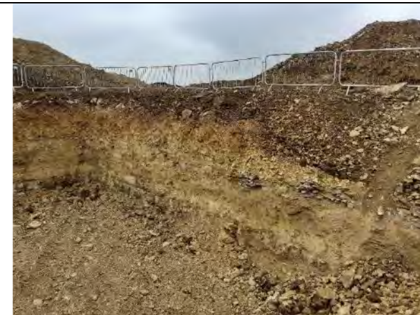
28.04.21 – Sidewalls and base absent from staining or indicators of fuel contamination
