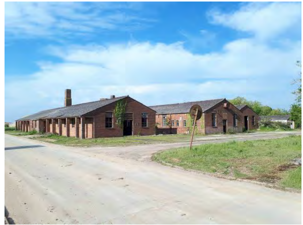
22.05.18 – Building's present across centre of the site
