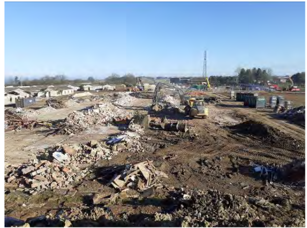
09.03.21 – Building demolition complete in the northern part of the site, recovery of hardstanding for processing
