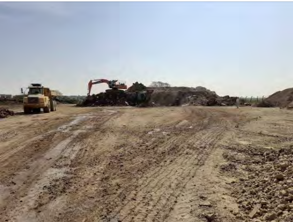
20.04.21 – Aggregate processing on-going
