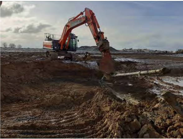
09.02.21 – Removal of pipeline from remediation excavation
