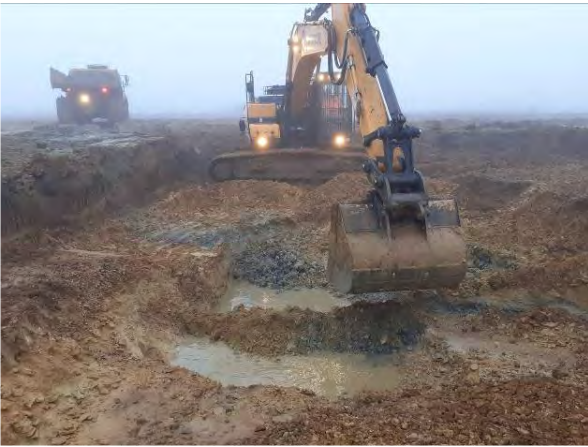
04.02.21 – Removal of clean overlying soils continued south down to impacted soils
