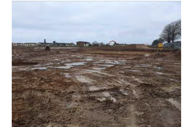
02.02.21 – View across baseball pitch following stripping and recovery of topsoil
