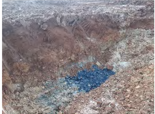
03.02.21 – Hydrocarbon impacted gravel evident by black colouration
