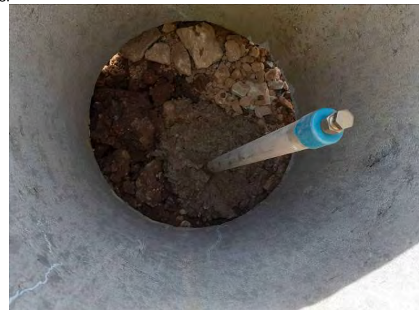
06.04.21 – Vapour probe installed within footprint of remediation excavation
