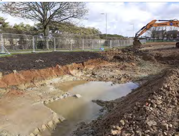
18.02.21 – Northern extent of hotspot remediation prior to backfill
