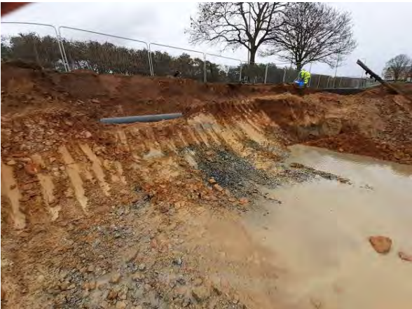
17.02.21 - Residual pocket of impacted soil awaiting removal
