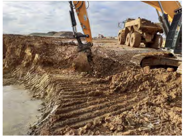
10.02.21 – Recovery of clean surface soils
