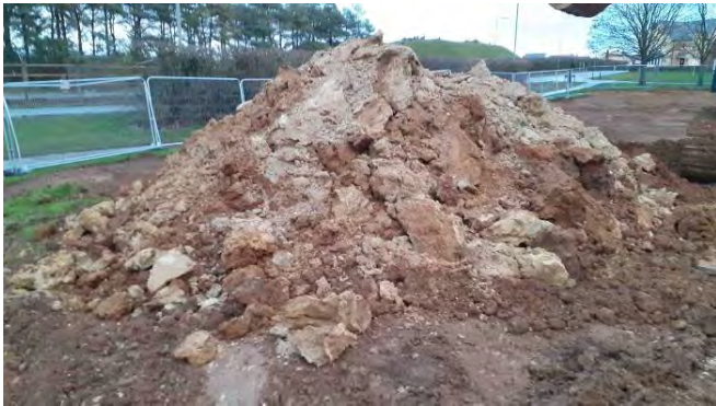
14.01.21 – Clean soils temporary stockpile to allow inspection
