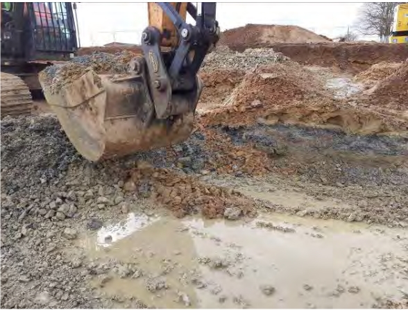
16.02.21 – Black / dark grey soils above bedrock shown thickness of impacted soil horizon
