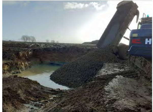
03.02.21 – Backfill of remediation excavation with aggregates
