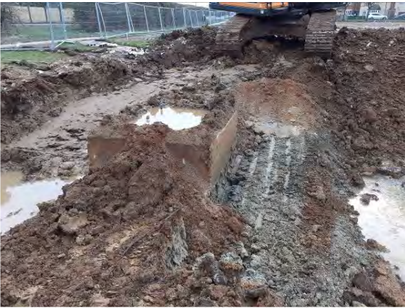
10.02.21 – Relict manhole chamber within northeast where impacted soils thin out.
