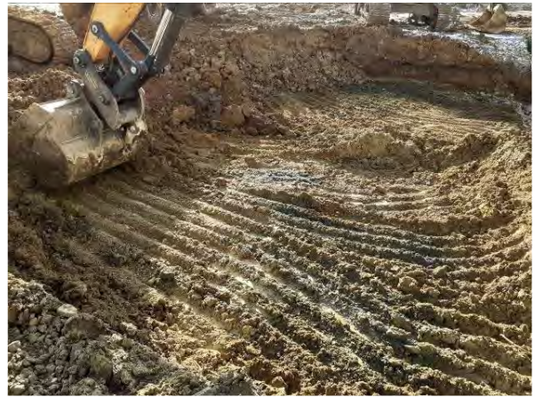
09.02.21 – Removal of clean surface soils from remediation area
