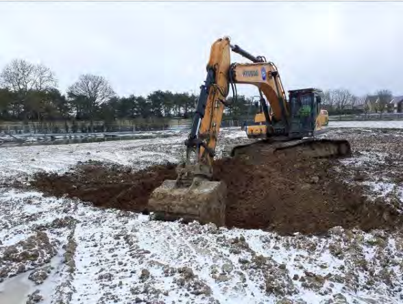
08.02.21 – Recovery of clean overlying soils from hotspot area
