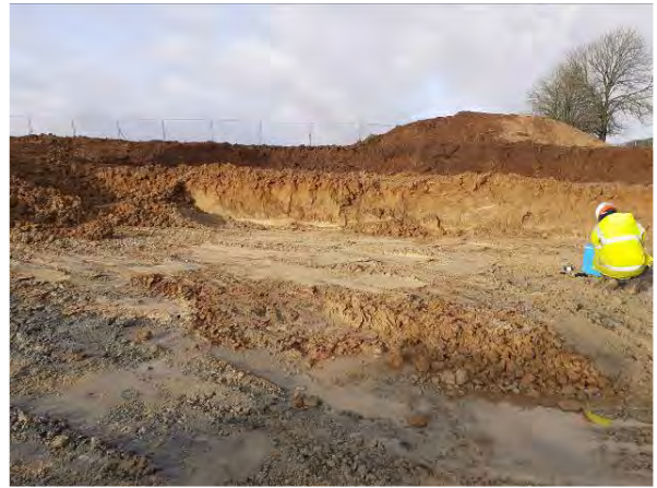
17.02.21 – Collection of validation samples at the base of the remediation excavation
