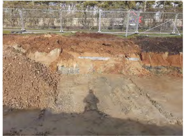
18.02.21 – Impacted soils appear to extend north towards Camp Road beyond the accessible extent of remediation
