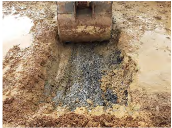
02.02.21 – Hydrocarbon impacted soils present as dark grey to black gravel beneath clean light brown soils/gravels.
