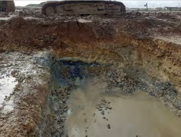
02.02.21 – Horizon of impacted soils visible approximately 1-1.5m below ground level
