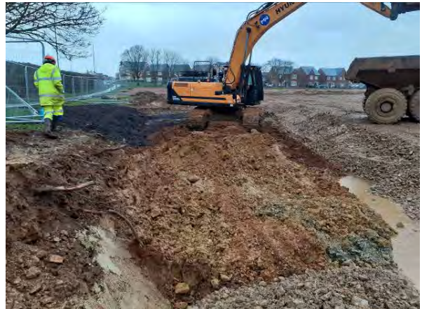
18.02.21 – Removal of clean overburden from northern extent of remediation excavation
