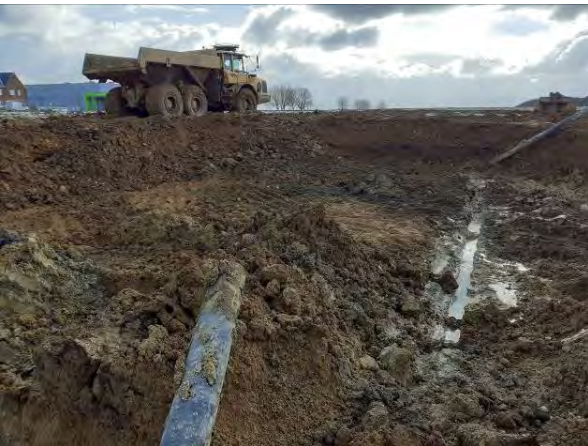
09.02.21 – Northeast extent of remediation excavation
