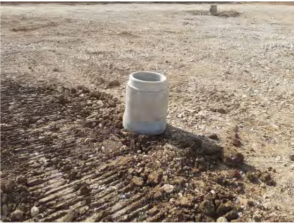
06.04.21 – Concrete collars placed over monitoring probes to protect during monitoring period
