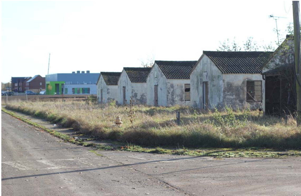
Figure 5: Looking east from Phase 9 at former school buildings.
