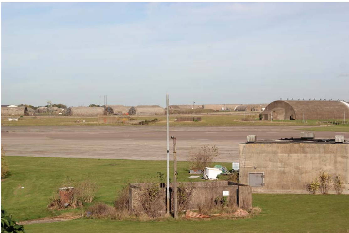
Figure 22: Looking towards the former Upper Heyford air base runways from the top of POL 21.
