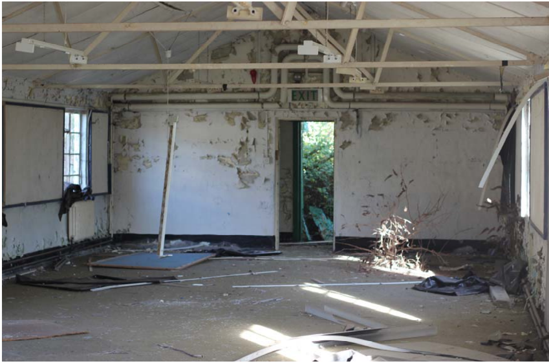
Figure 13: Looking within one of the former school classrooms.
