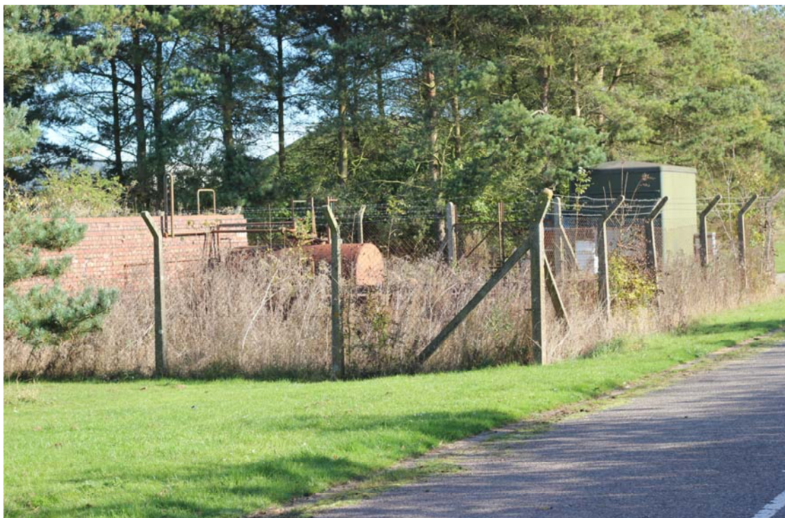
Figure 16: Looking at above ground tanks in Phase 10.
