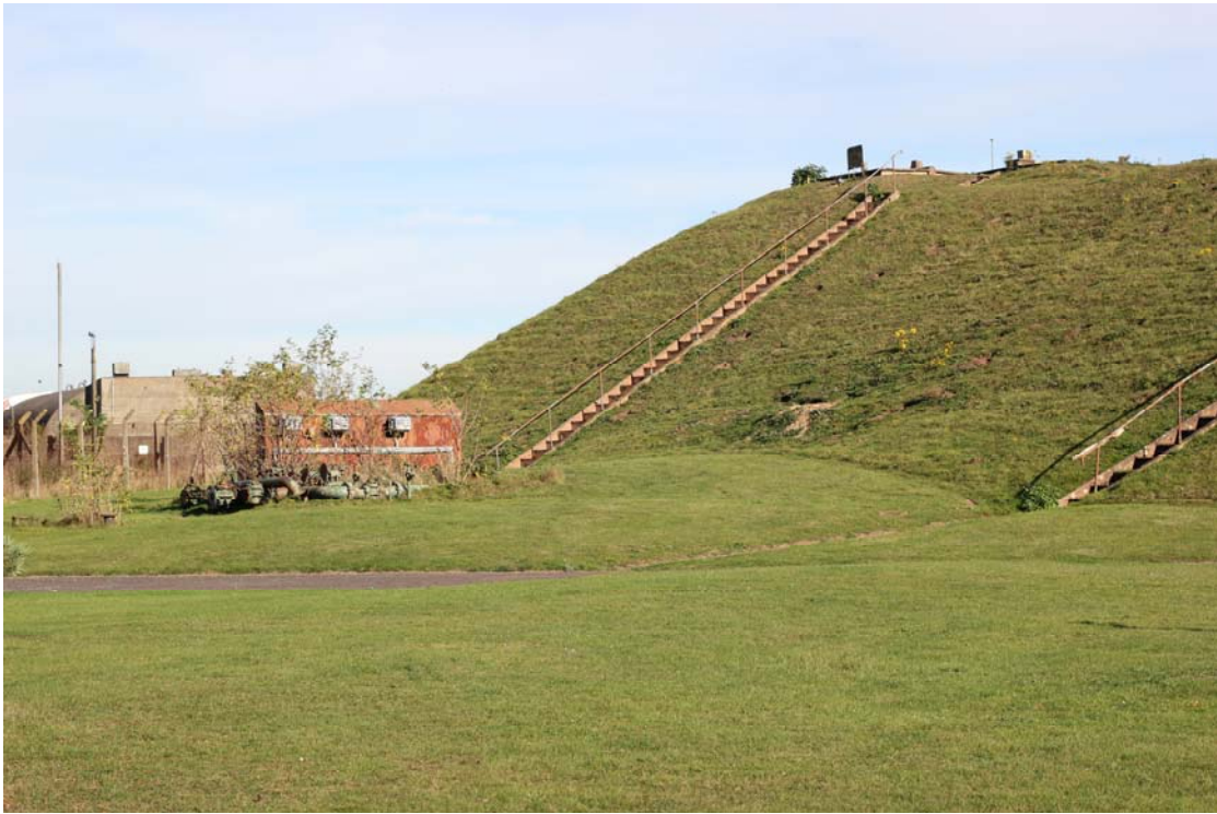
Figure 19: Looking north towards POL 21.
