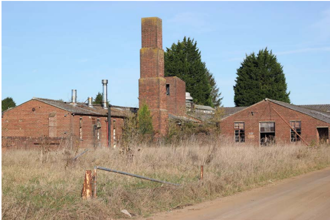
Figure 9: Looking at former boiler house on Phase 9.
