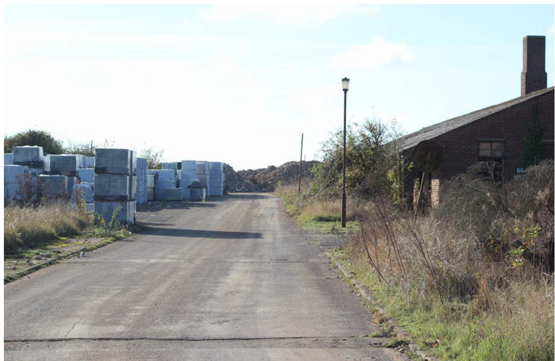
Figure 6: Looking south from Phase 9. Note, boiler house to right of shot, stockpiles breeze blocks to left of shot and concrete stockpile in distance.
