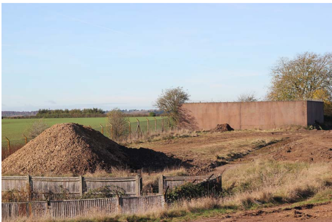
Figure 12: Looking at tanks in southeast of Phase 9. Note, tanks in the foreground and in the background of shot.
