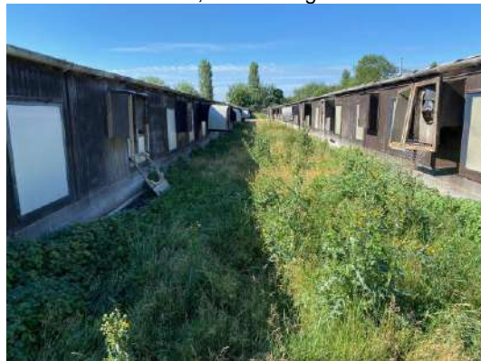
View facing south between two former chicken sheds
