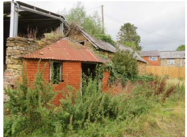
Figure 14. the south-west elevation of the outbuilding (Figure 3: B2)
