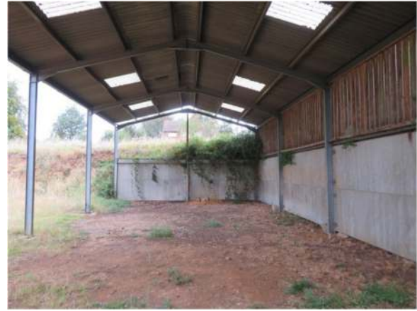
Figure 18. The interior of the steel-framed barn
