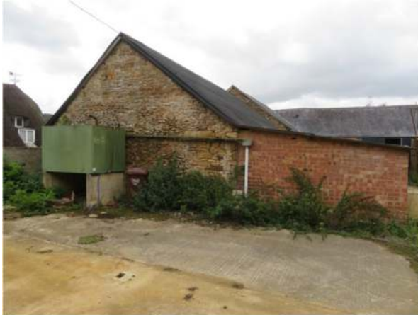
Photograph 1. The east elevation of the southern part of the L-shaped barn
