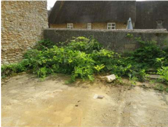
Photograph 24. Concrete area at the south-east corner of the site
