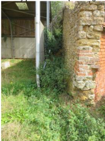
Photograph 28. Wall to the rear of the outbuilding
