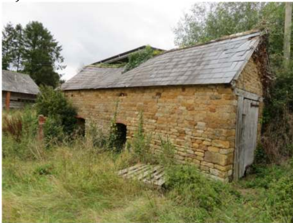
Figure 13. The south and east elevations of the outbuilding (Figure 3: B1)
