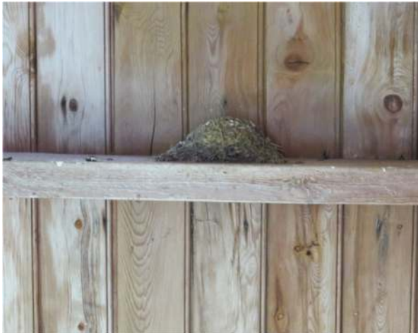
Photograph 33. Swallow's nest in the northern section of the western part of the L-shaped barn (Figure 3: A1)
