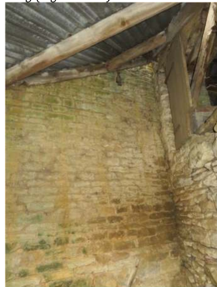
Figure 16. The interior of the south-west corner of the outbuilding (Figure 3: B2)
