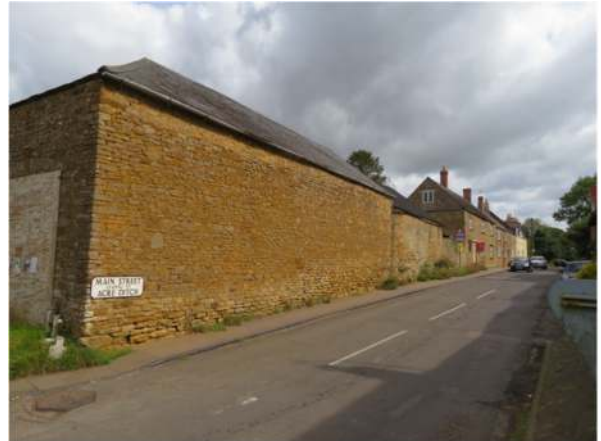
Photograph 6. The southern elevation of the southern part of the L-shaped barn
