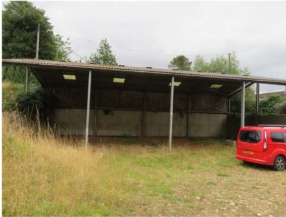
Figure 17. The west elevation of the steel-framed barn (Figure 3: C)
