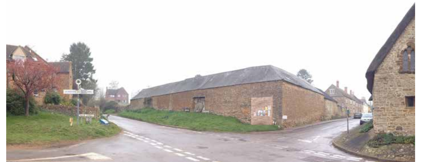
Fig. 16 - Mawles Farm on corner of crossroads between Main Street and Pound Lane
