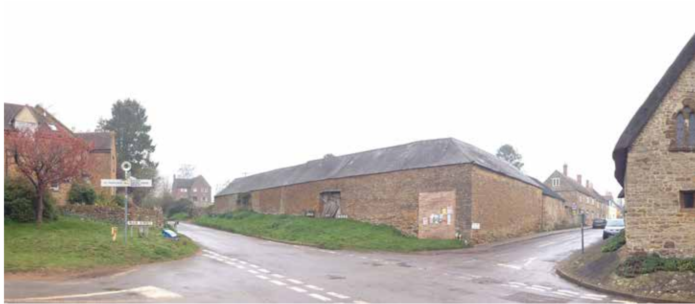
View 1 - Mawles Farm looking north from the crossroads
