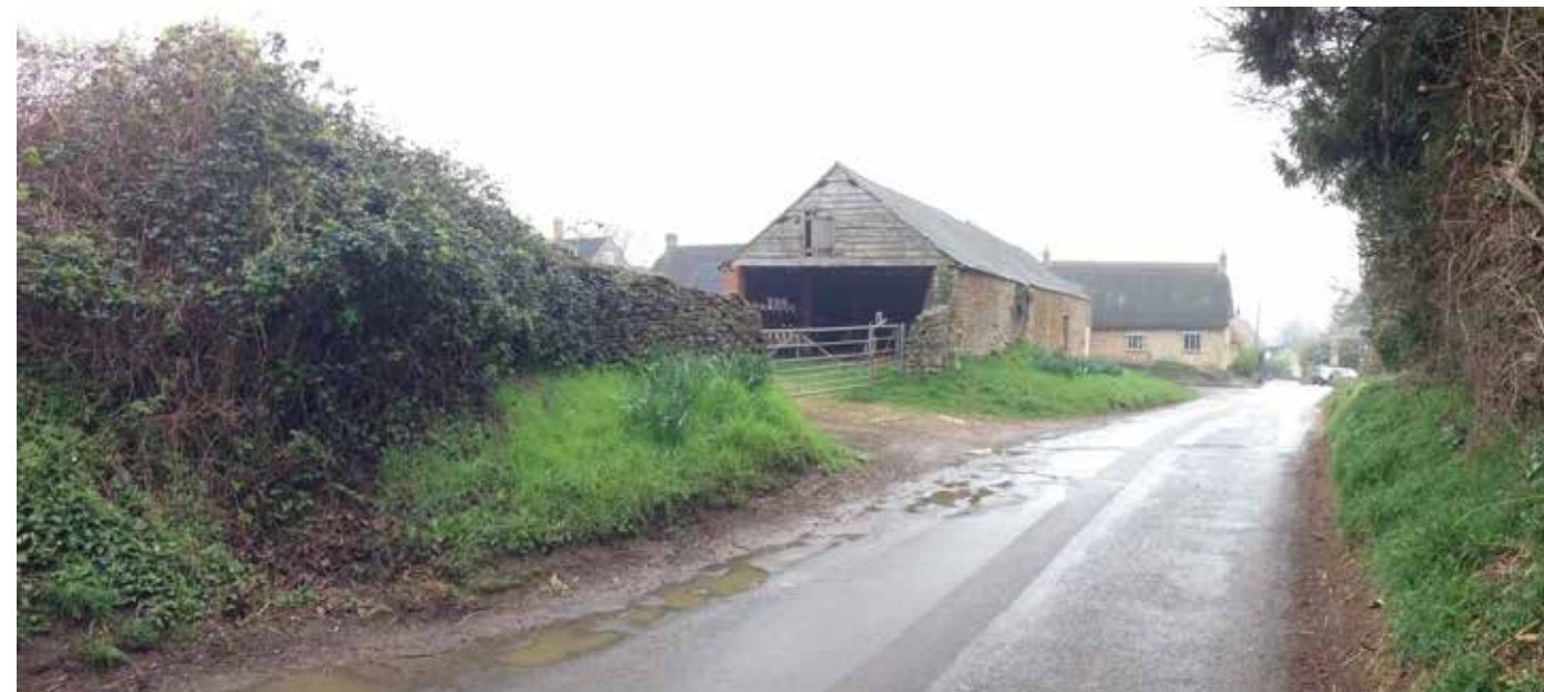
Fig. 14 - Approach to Mawles Farm looking south down Pound Lane
