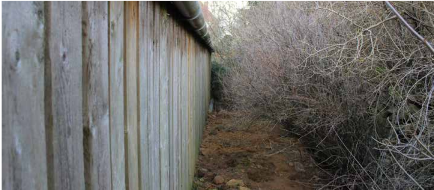
View 20 - Upper ground level area to the rear of the modern steel barn
