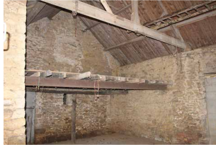
View 29 - Threshing barn interior with hay loft
