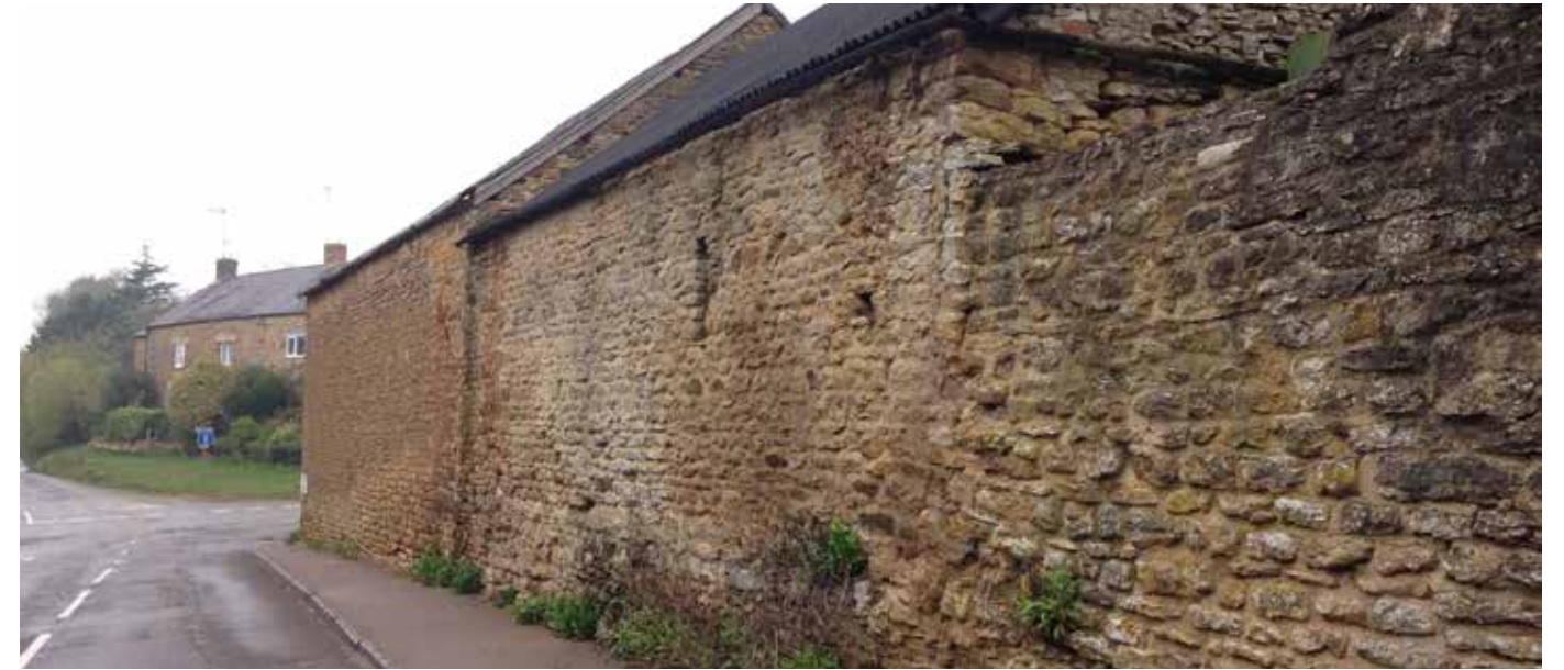
View 8 - Southern wall of Mawles Farm barns on Main Street
