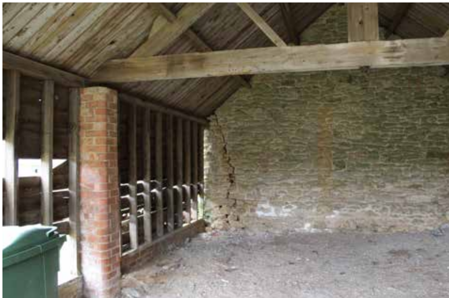
View 27 - Cart shed interior
