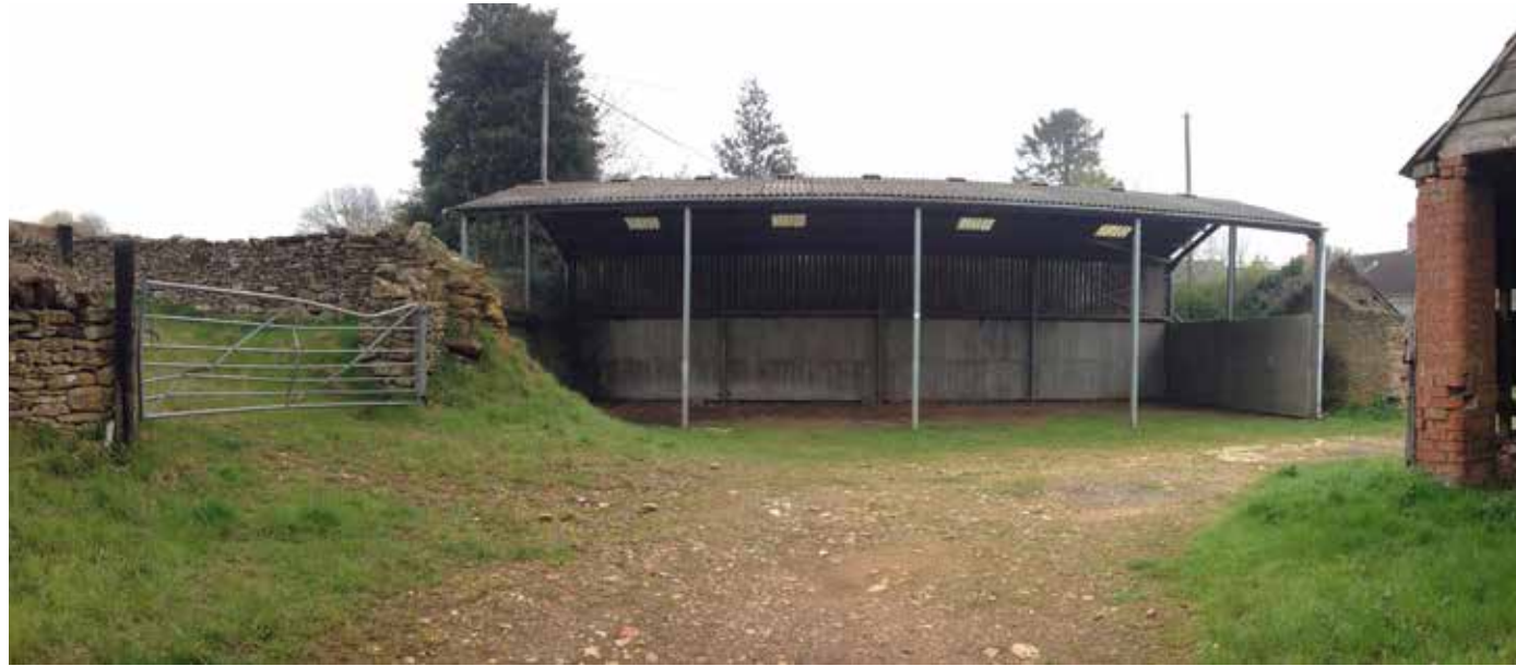
View 15 - Site entrance from Pounds Lane showing modern steel pole barn
