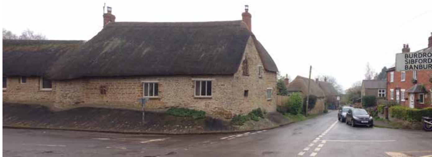
View 2 - Carter's Yard and Colony Road looking south from the crossroads
