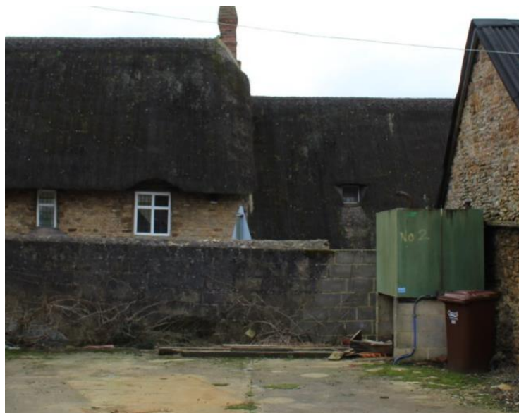
Photograph of wall to be rebuilt showing blockwork construction
