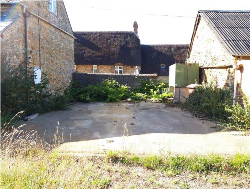
Photograph C: Looking south at the refuelling area, including fuel tank
