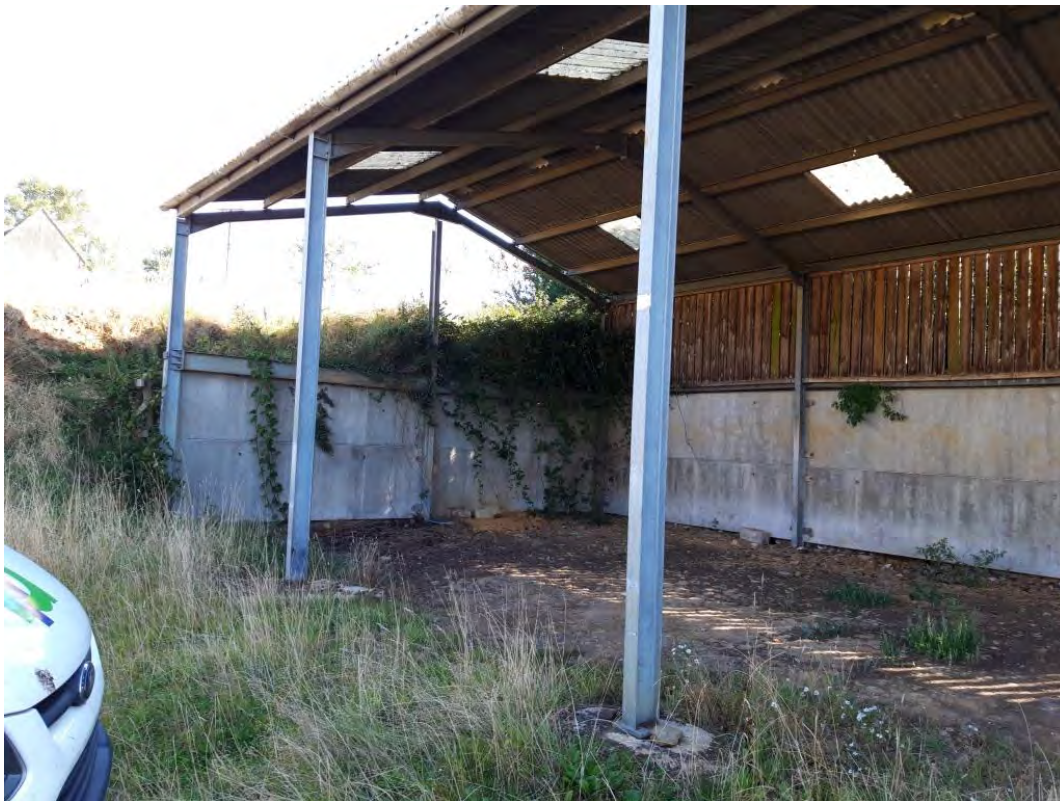
Photograph H: Looking northeast at the modern storage barn
