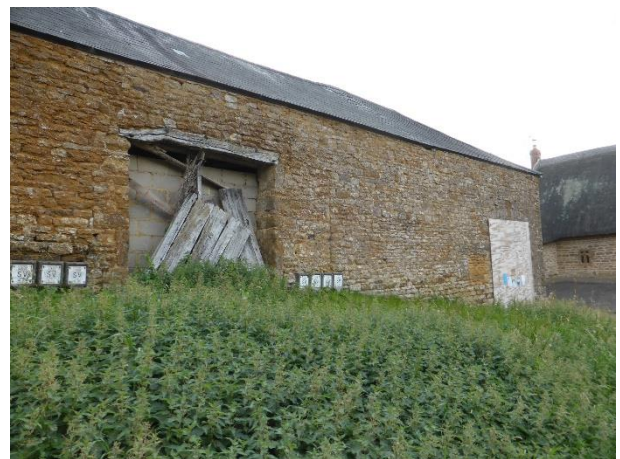
Blocked up opening
