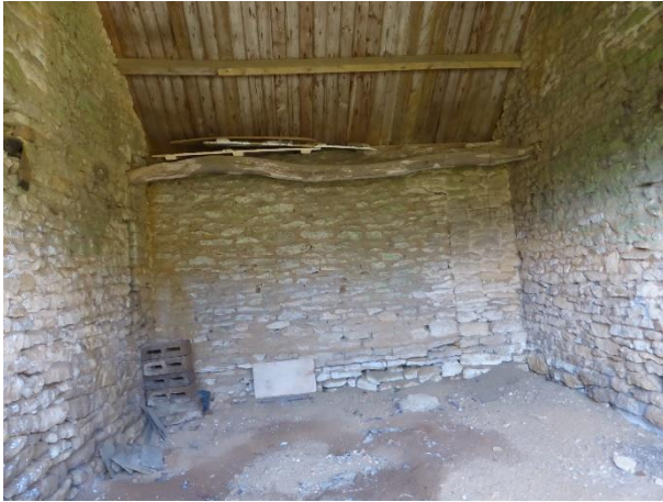
Drivethrough wall infilled
