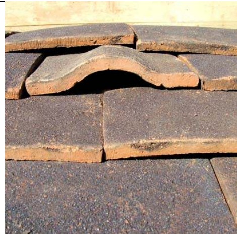
Photograph 2. Example of a bat access tile
