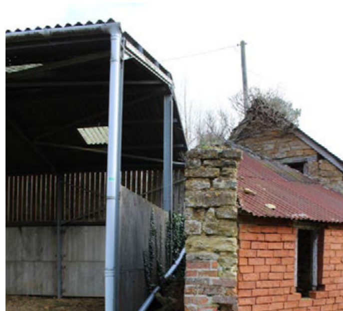
Fig. 26 - Steel pole barn and the piggery
