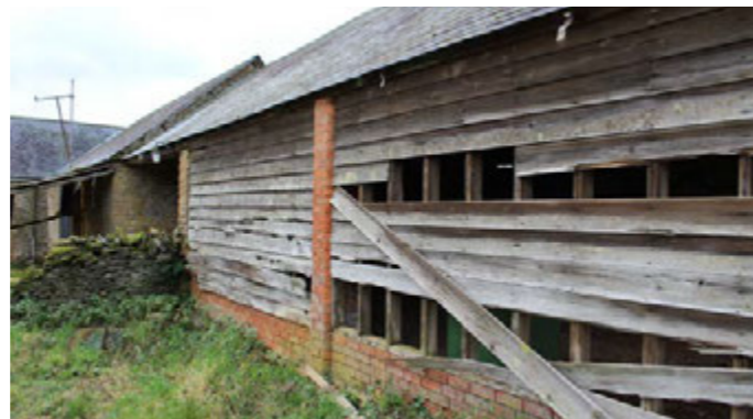
Fig. 15 - Brick and timber alterations
