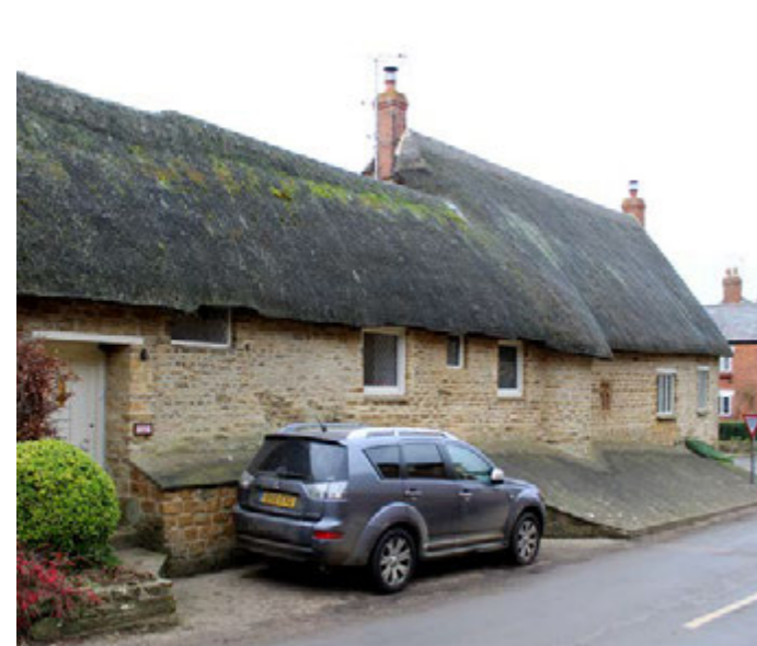
Fig. 23 - Carter Yard viewed from Main Street
