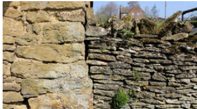
Fig. 14 - Coursed ironstone rubble and walling stone
