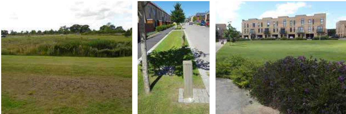
From left: attenuation pond, South West Bicester; swale, Trumpington Meadows, Cambridge; dry detention basin within parkland, Clay Farm, Cambridge.
