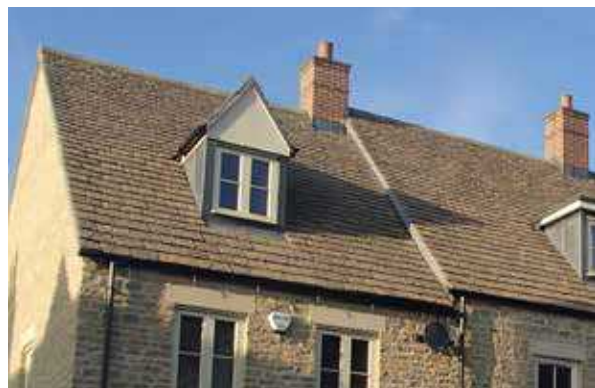
Good examples of modern dormer windows, pitched roofs, slate tiles and brick chimneys, Woodstock
