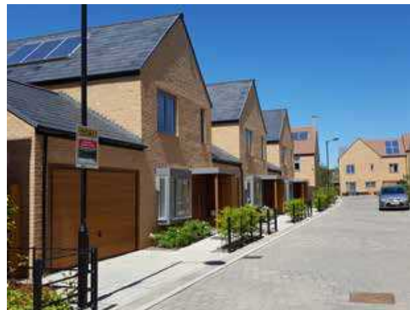
Photovoltaic panels, Trumpington Meadows, Cambridge
