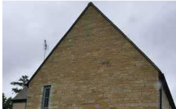
Steeply pitched roof with no overhang, Bletchington
