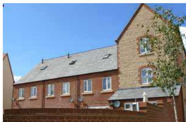
Small rooflights on rear elevation, South West Bicester
