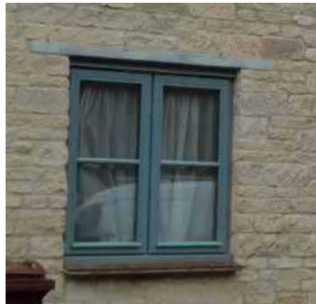
Casement window flush with wall, Bletchingdon
