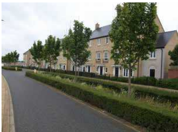
An avenue of tree and low hedges along Whitelands Way, South West Bicester is in keeping with the formal character of the street
