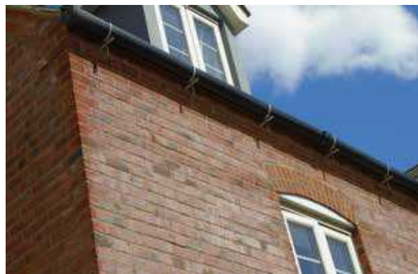
Guttering, South West Bicester
