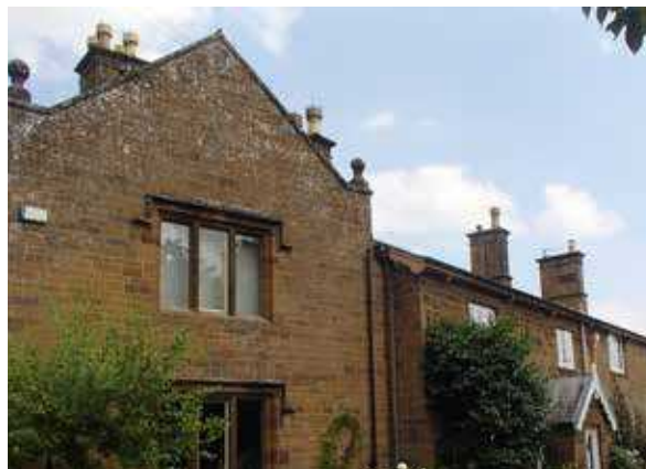
Two to three storey buildings, Adderbury
