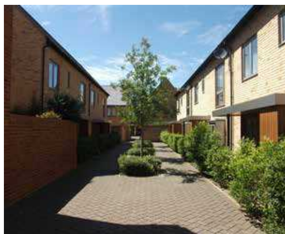
Mews street, approximately 7m wide, Trumpington Meadows, Cambridge
