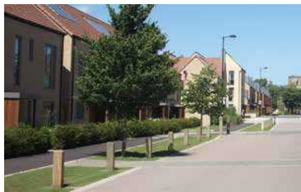
Incorporating SuDS along kerbside, Trumpington Meadows, Cambridge
