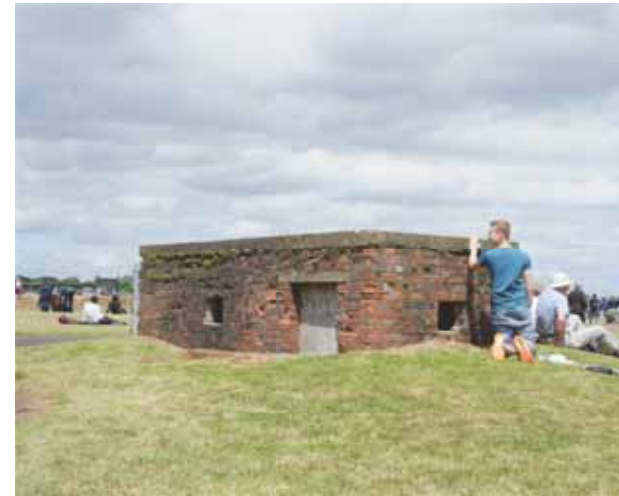
ABOVE A retained air raid shelter at Bicester Heritage creates a natural gathering point during events, its shadow offering some welcomed shade on hot summer days. Photo taken at RAF Bicester Heritage, Bicester, 2016 © of GHVDC Ltd
