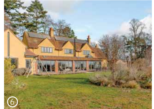
Existing Dwelling House
