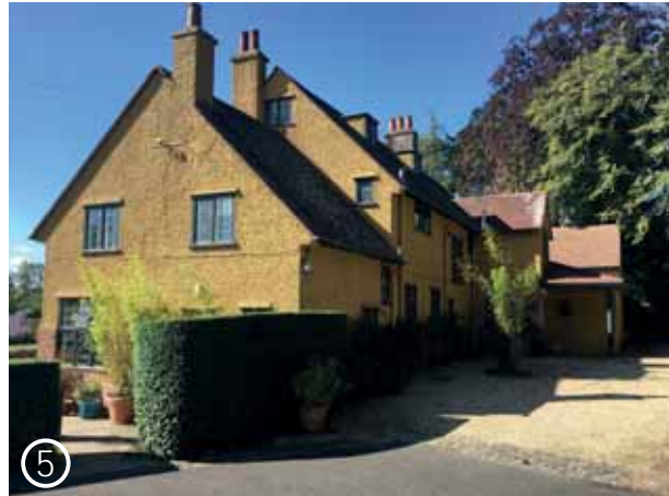
Existing Dwelling House
