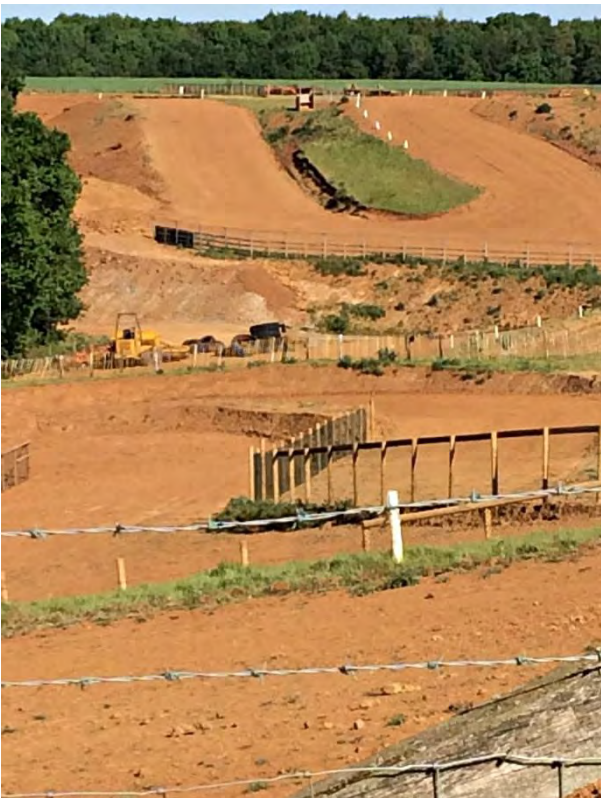
Left: the resulting track after major circuit works in May 2020
