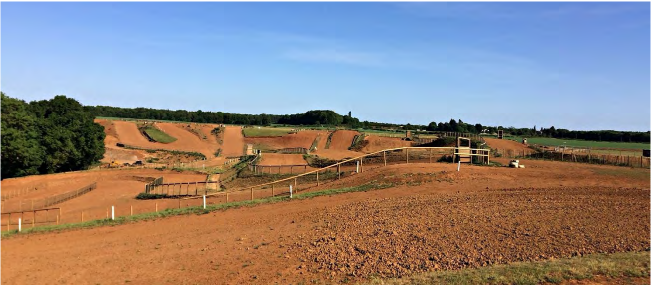
Above: After further earthworks during Covid lockdown, May 2020 (Photos this page: Hornton villager)
