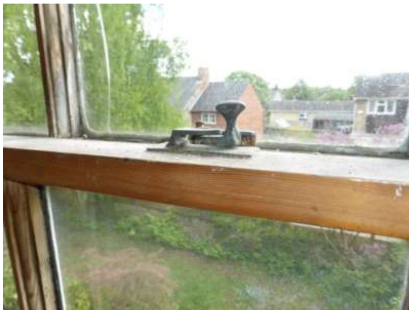
Figure 41: Later 19 th to early 20 th century window details in F1
