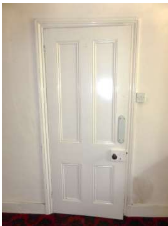
Figure 21: An early 20 th century door and architrave between G1 and G2
