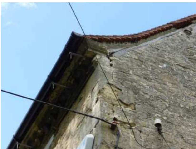
Figure 7: Bellcast eaves and stone quoin details
