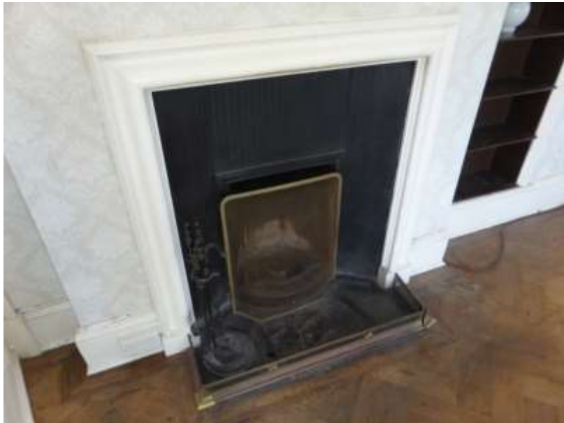
Figure 50: Early 20 th century coal grate with bolection moulding surround
