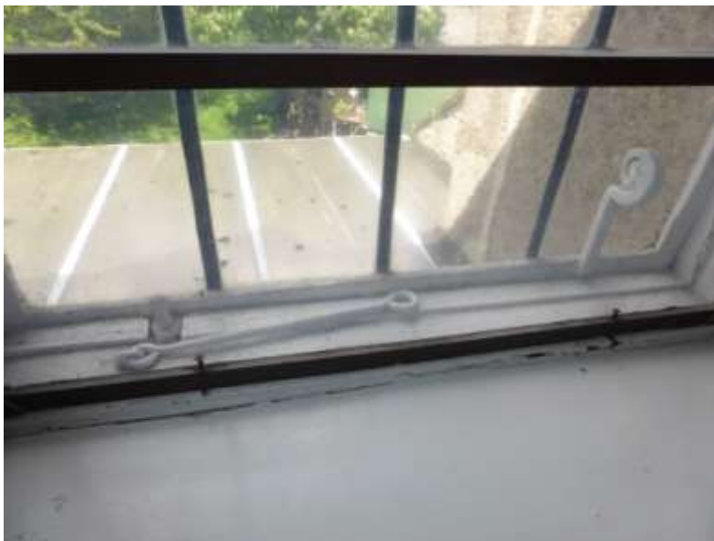
Figure 47: Casement handle and stay in F3
