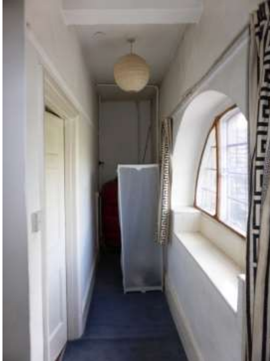
Figure 42: Rear section of F2 with early 18 th century thermal window to the right
