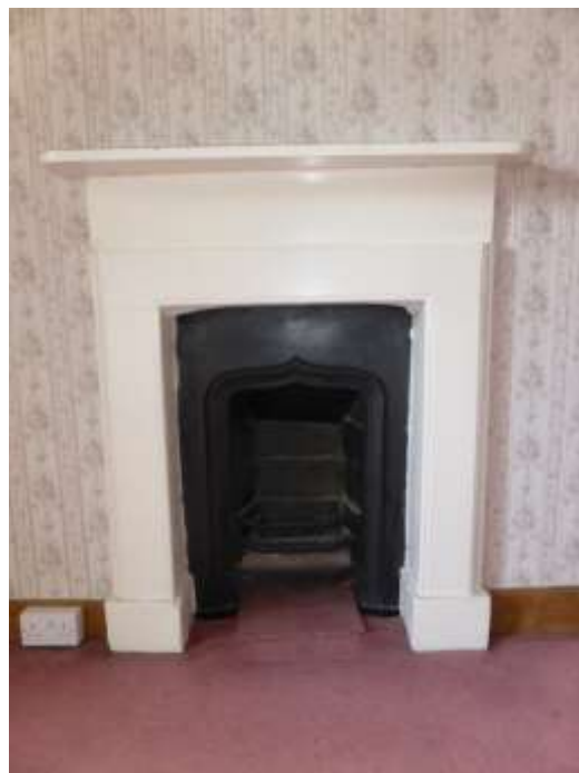
Figure 39: Later 19 th century coal grate in F1
