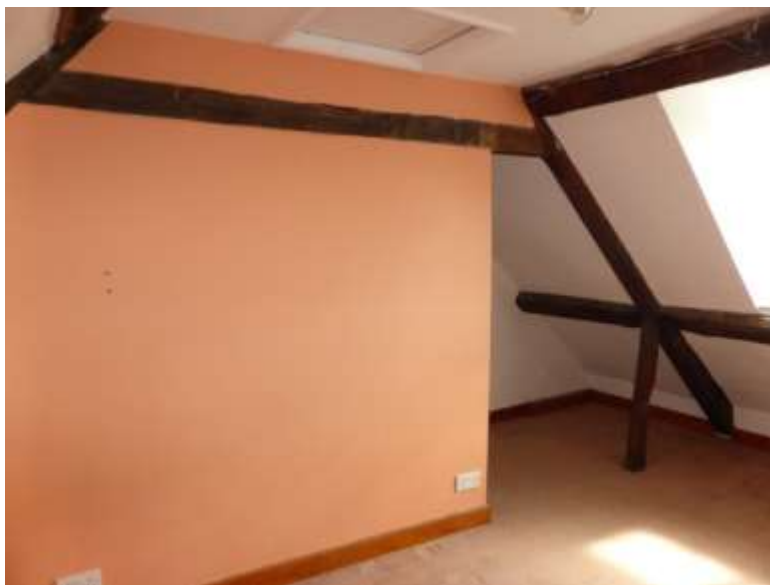
Figure 54: Collar truss in A1
