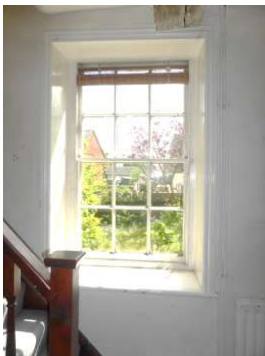
Figure 23: Six over six sash window in G1 with chamfered glazing bars and later 19 th century style fastener
