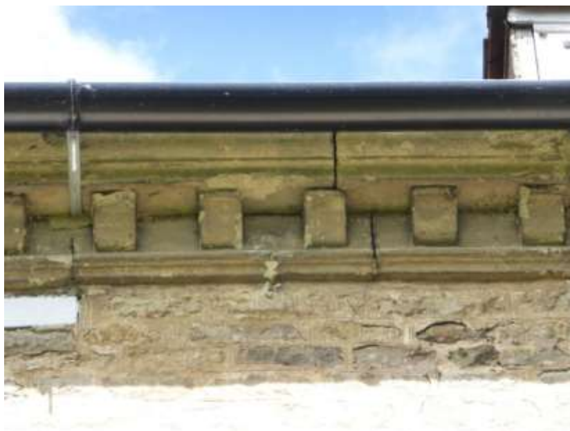
Figure 6: Stone dentil cornice
