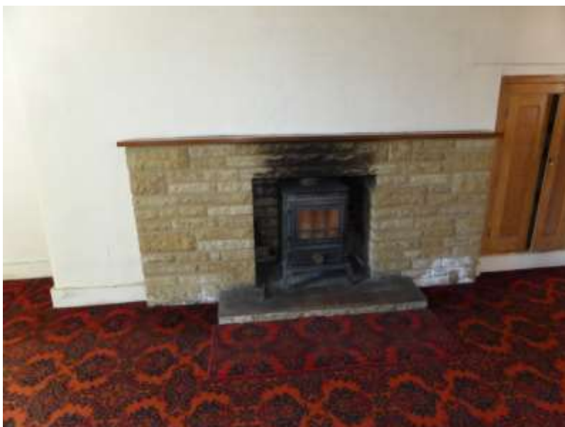
Figure 24: Modern fireplace in G1
