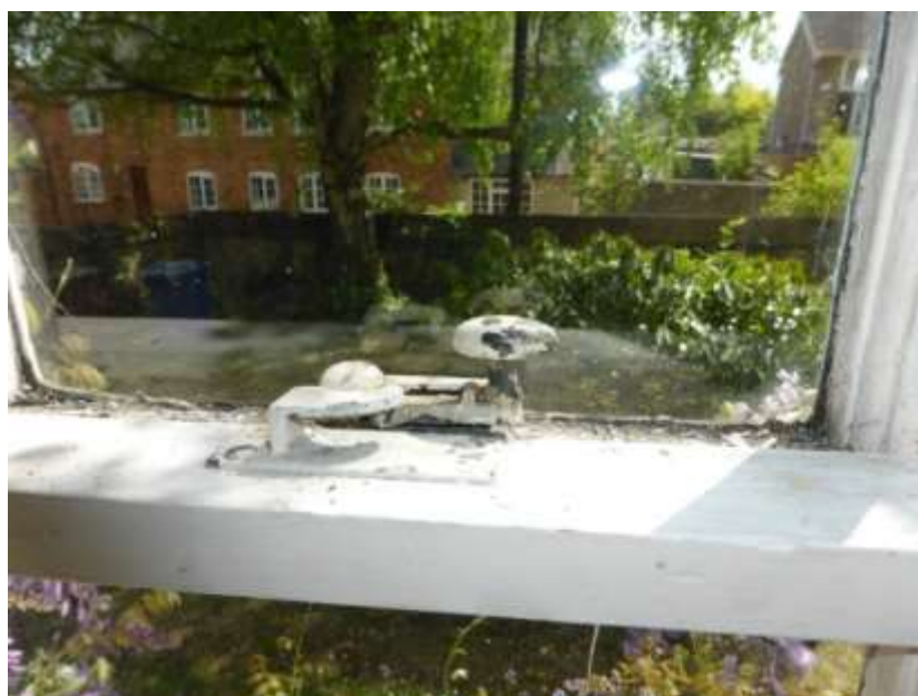
Figure 30: Late 19 th century style sash fastener in G6
