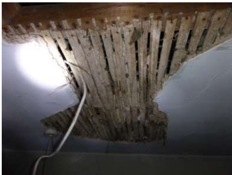
Figure 36: Lath and plaster ceiling above the modern ceiling
