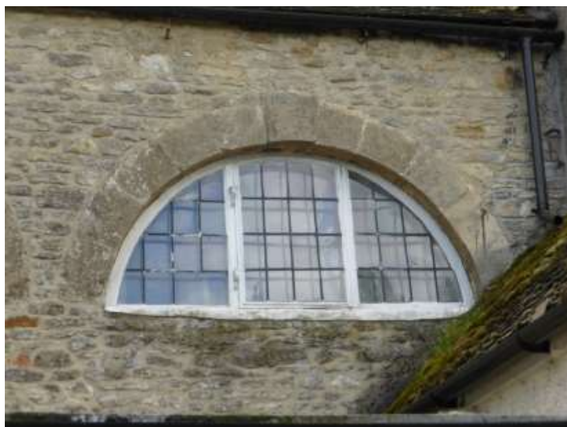
Figure 14: Detail of the early 18 th century thermal window on the right hand side
