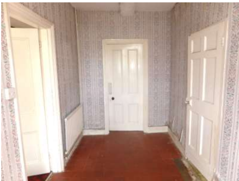
Figure 25: The Hall (G2) looking north
