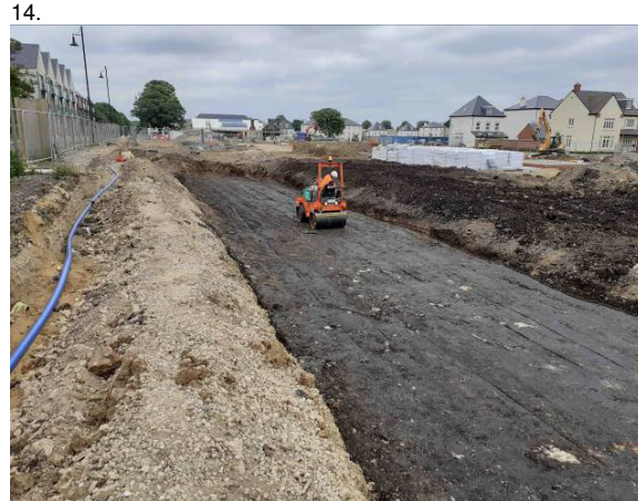
08.06.20 – Retained soils replaced and compacted into Phase 4 excavation.
