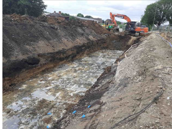
04.06.20 – View west across excavation area.
