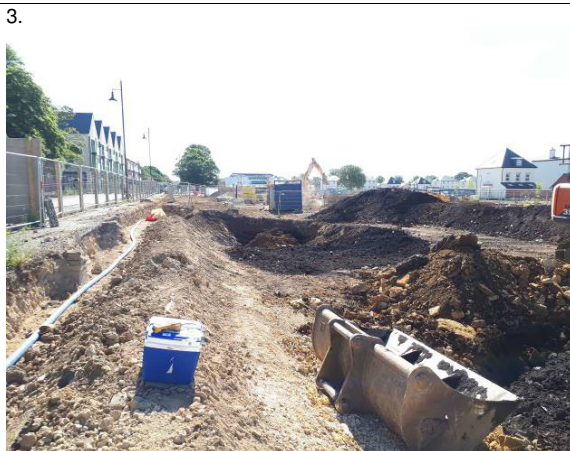
02.06.20 – Eastern view down remediation area (Camp Road visible to left)
