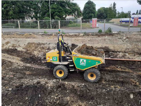
04.06.20 – Removal of contaminated soils to quarantine area within wider development.
