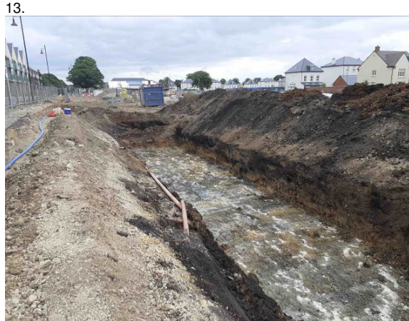
04.06.20 – View east across excavation area.
