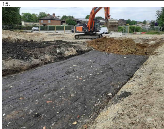
08.06.20 – Continuation of excavation to west
