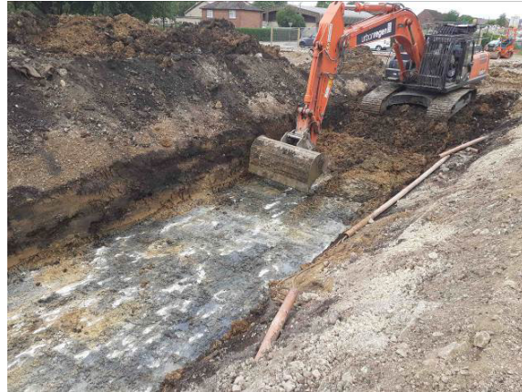
04.06.20 – Continuation of excavation of hydrocarbon contaminated soils down to weathered bedrock.
