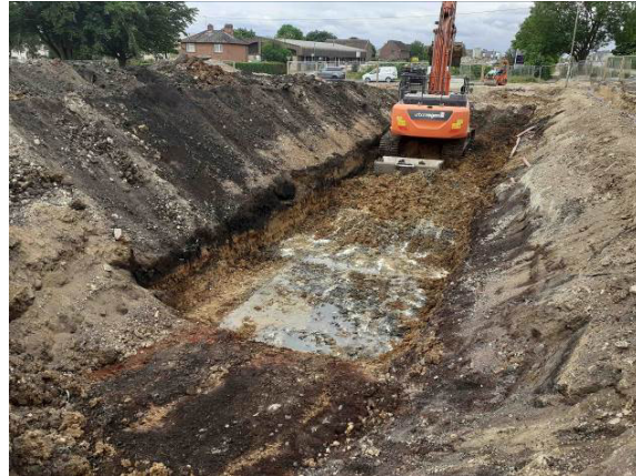
04.06.20 – Excavation of hydrocarbon contaminated soils down to weathered bedrock.
