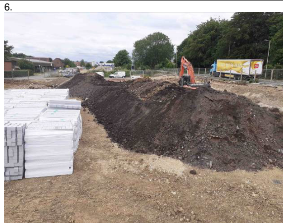
04.06.20 – Soils not demonstrating significant contamination indicators stockpiled to south of excavation area (1/2).
