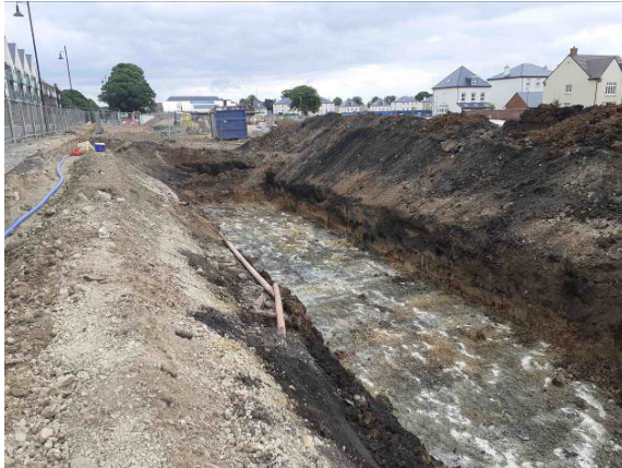
04.06.20 – View east across excavation area.
