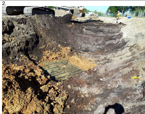
02.06.20 – Clean stone removed from surface exposing impacted clay soil at base
