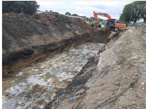
04.06.20 – View west across excavation area.
