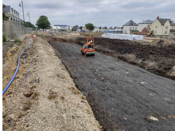
08.06.20 – Retained soils replaced and compacted into Phase 4 excavation.
