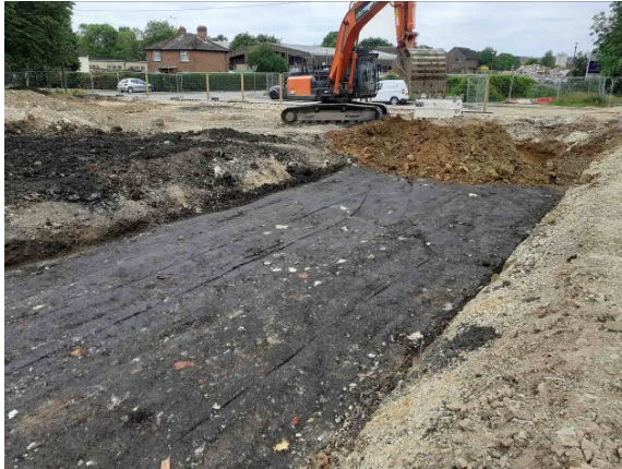
08.06.20 – Continuation of excavation to west
