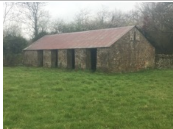
Photo 3: The southern elevation of the barn
