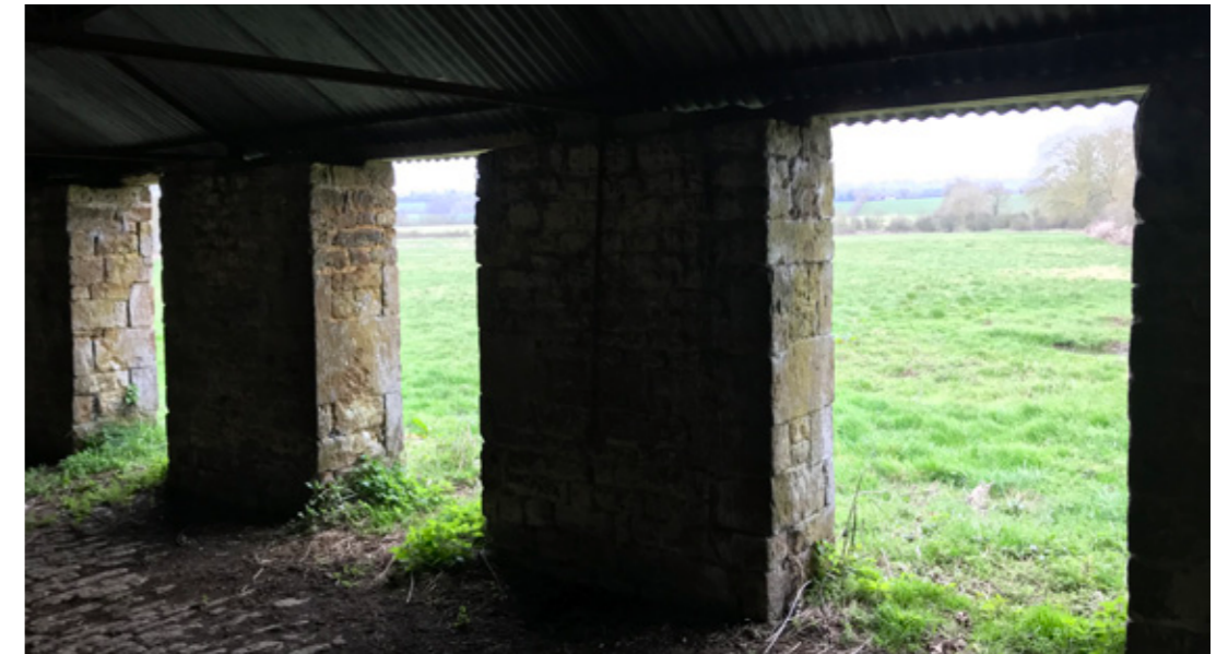
Barn windows frame long distance views into meadow and hedgerow.
