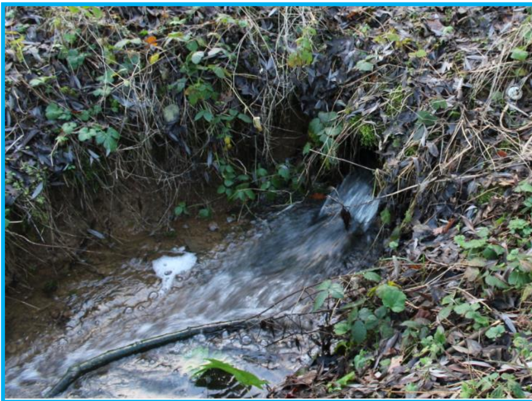
Fig 16 300mm outlet from pond into watercourse indicating inlet blocked (pond was overflowing).
