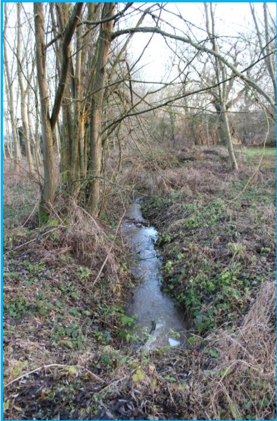
Fig 17 Well-defined outlet channel from pond, approx. 600mm wide bed with sloping banks and 600mm deep (as on survey).
