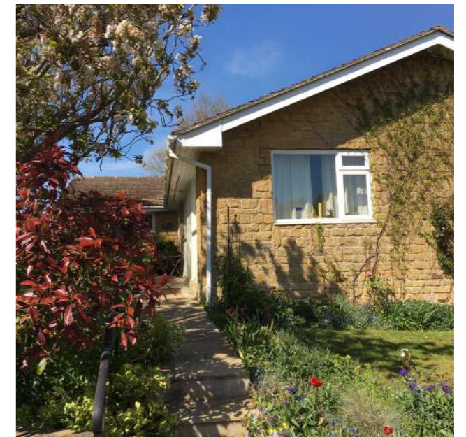
6. View of the south elevation
