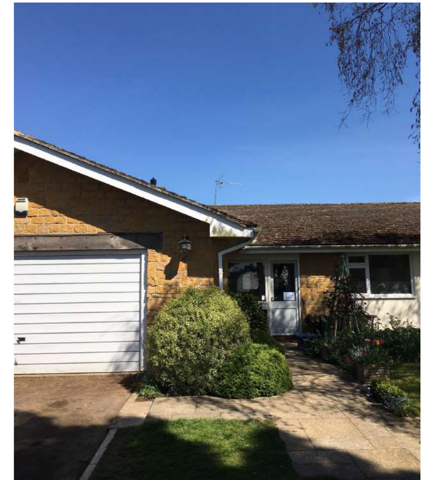
3. View of the existing garage and the front porch
