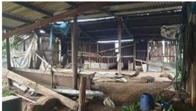
Figure 2 – timber lean-to which will be demolished
