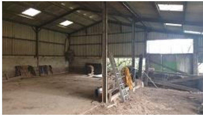
Figure 1 – internal view into the appeal building
