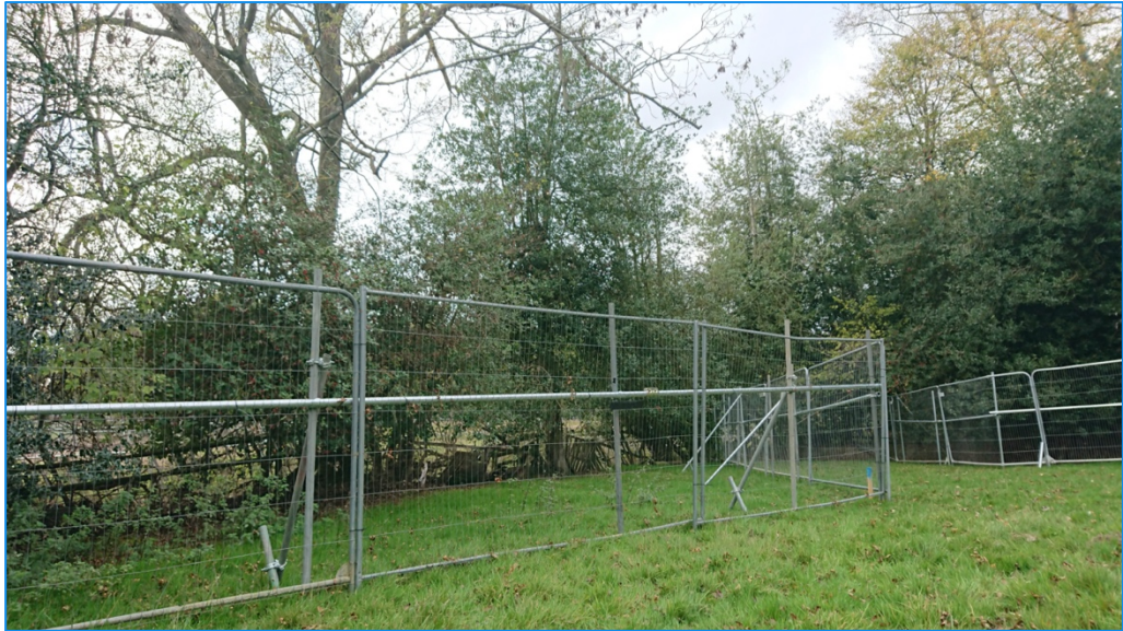
Typical tree protection barrier construction
