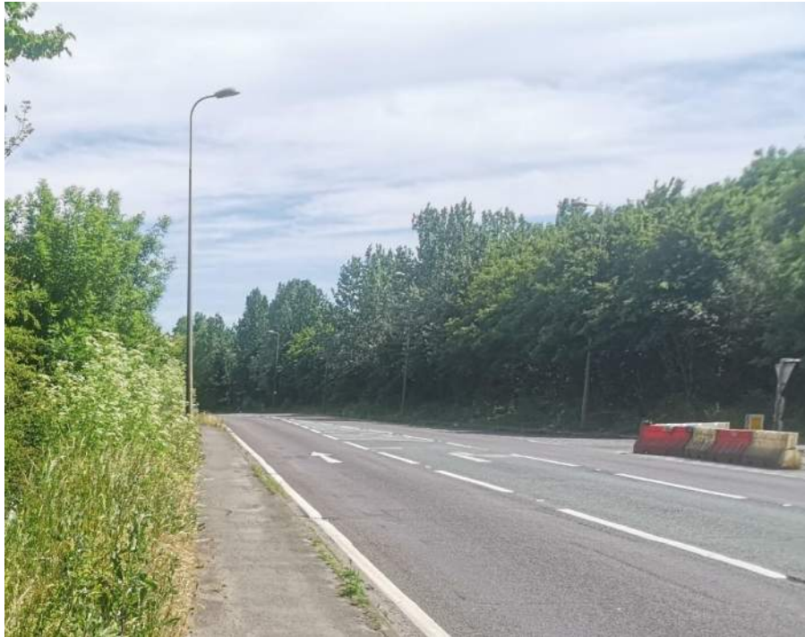
Photograph 3 – Roads and pavements within the Site.
