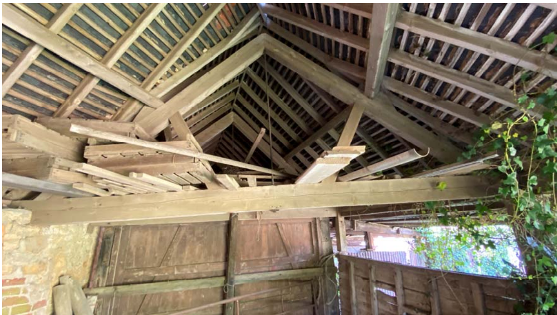
Typical Principle truss and purlin arrangement in hovel
