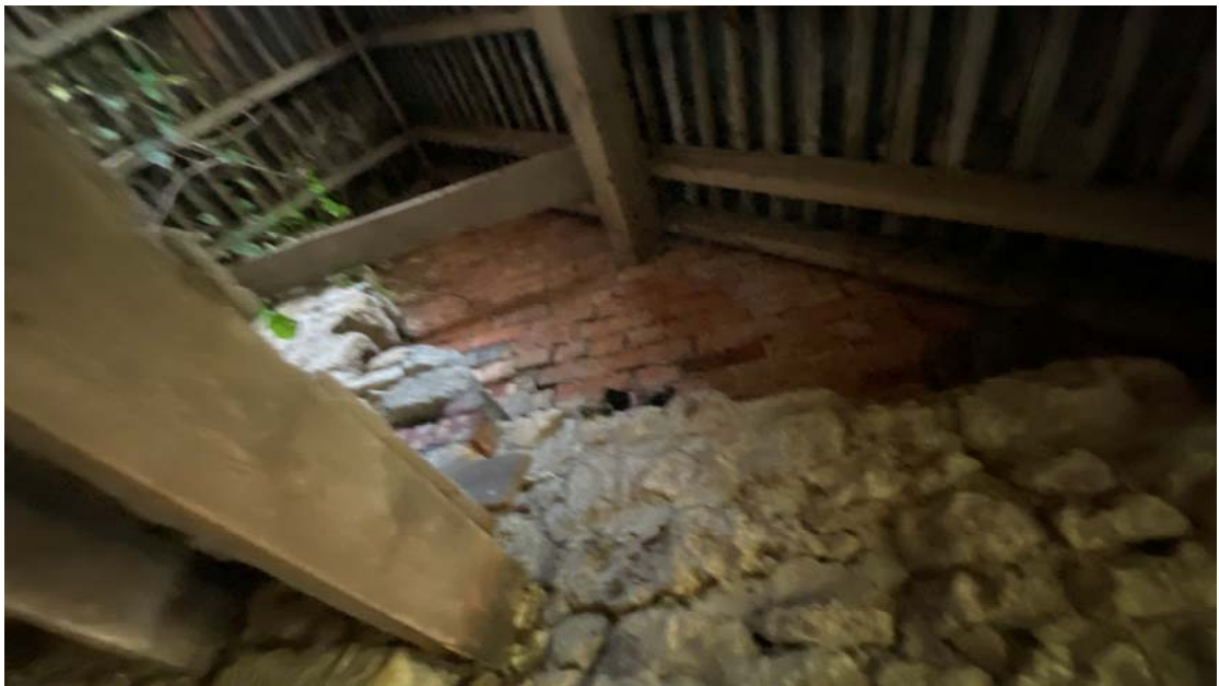
Mixture of stone and brick gable to Northern section
