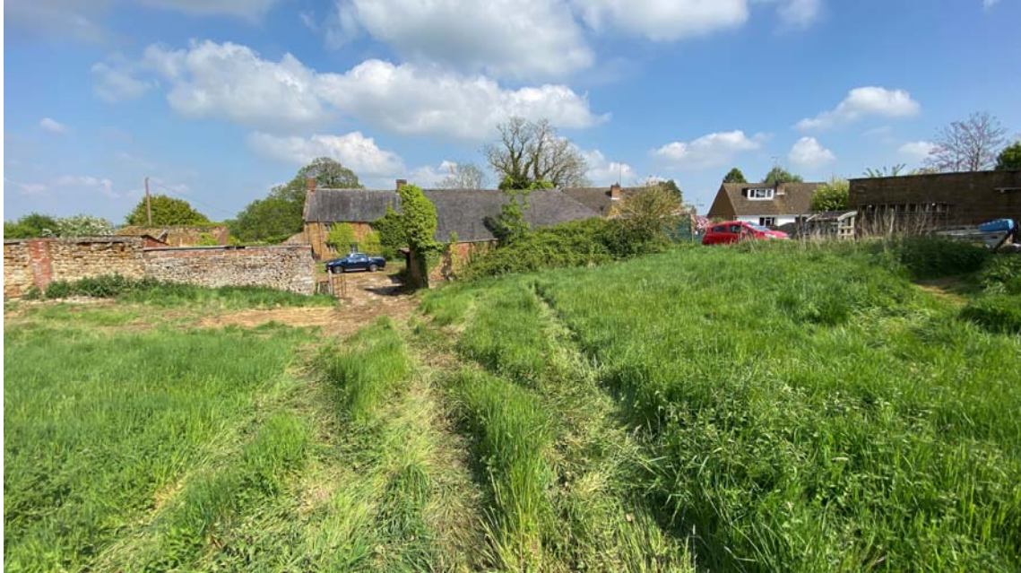
Northern Elevation showing neighbouring driveway and retaining nature of rear wall
