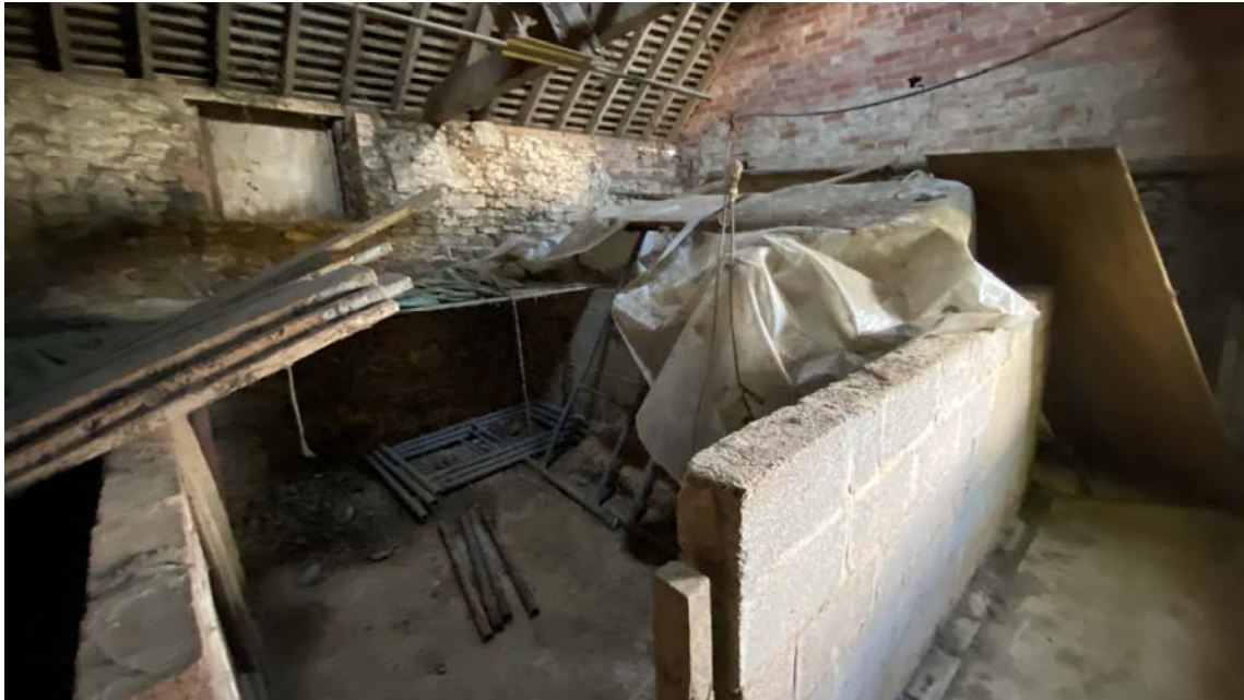
Northern section of the buiding with block walls to waist height.
