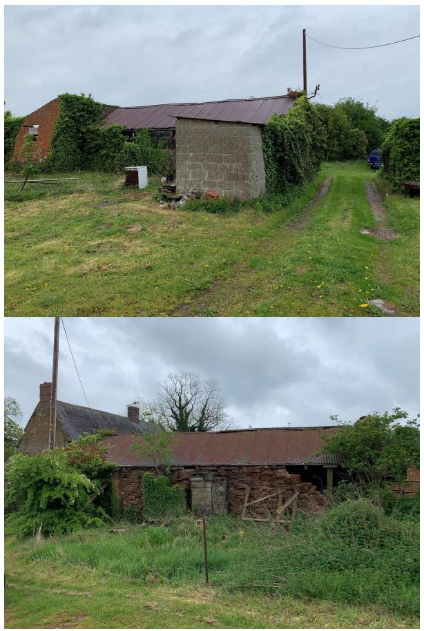
Figure 17: Buildings 7 and 8, front (top) and rear – note the very poor condition of the back wall.
