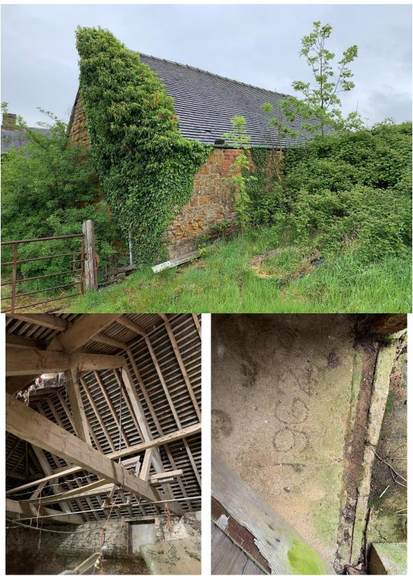
Figure 14: Views of building 4 - top, the rear (west) elevation showing ironstone ashlar construction but with some rebuilding in brick; bottom left, the late  $19^{th}$ /early  $20^{th}$ -century roof trusses and modern roof covering over them; bottom right, the date 1962 in the concrete floor. Vegetation is engulfing this elevation – compare with Soden 2016, figure 9.
