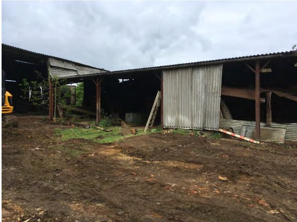
Photo 1: The site looking northwest showing the northernmost barn and northern courtyard.
