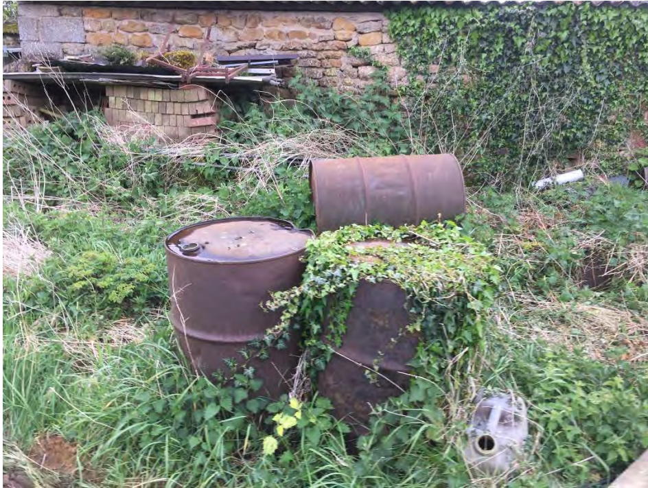
Photo 7: Multiple unlabelled empty/water filled drums in the east of the site.
