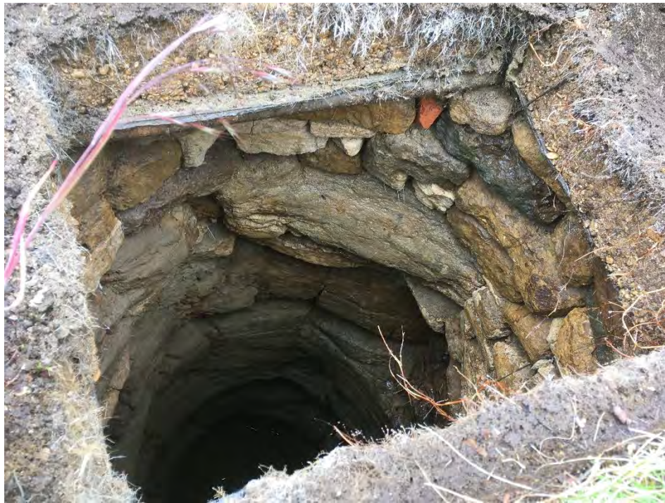
Photo 9: Well chamber is located to the centre of the site.
