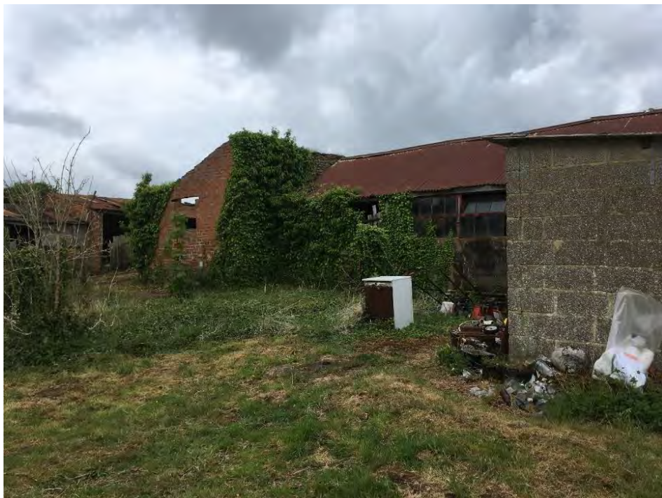
Photo 2: The site looking northwest showing the southern courtyard and dilapidated barns.
