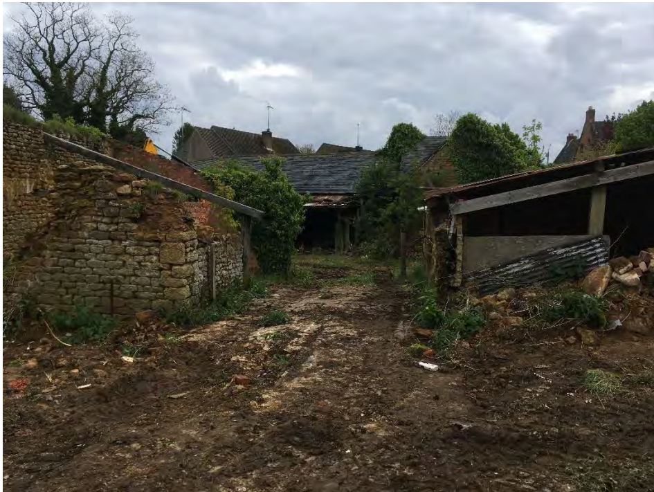
Photo 4: The site south showing the dilapidated farm buildings.
