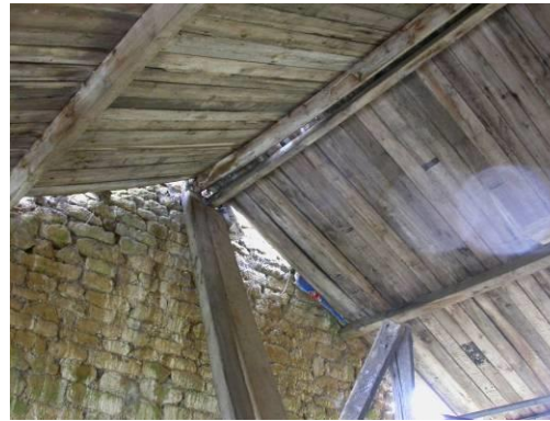
Figs. 18 & 19 Timber sarking lined roof of stable block
