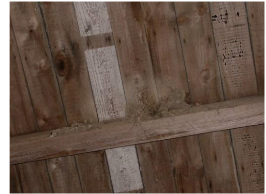
Figs. 18 & 19 Timber sarking lined roof of stable block
