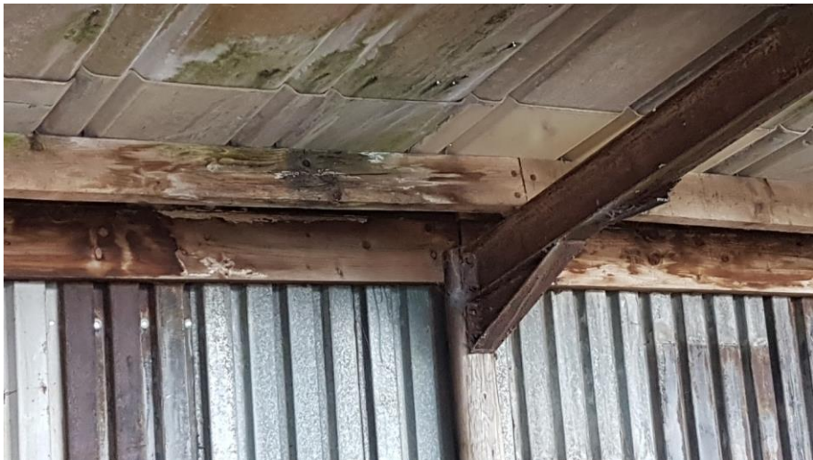
Connection between steel rafter and timber column
