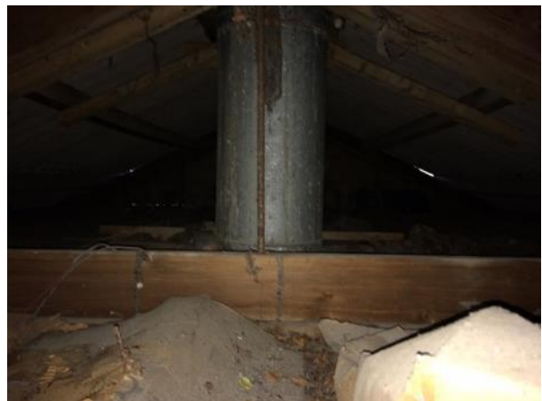
Photograph 6. The loft space within the southern section of Building D.
