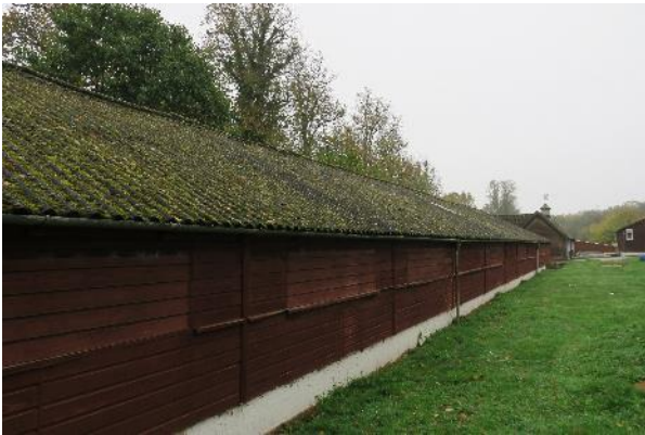
Photograph 3. Building C viewed from the north-west.
