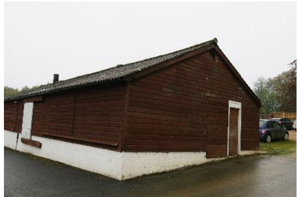
Photograph 4. Building D viewed from the north-west.
