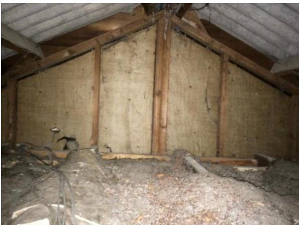
Photograph 5. The loft space within the northern section of Building D.
