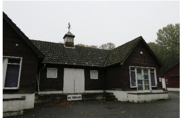
Photograph 8. Building F viewed from the east.
