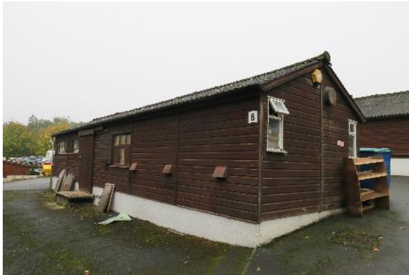
Photograph 7. Building E viewed from the north-east.
