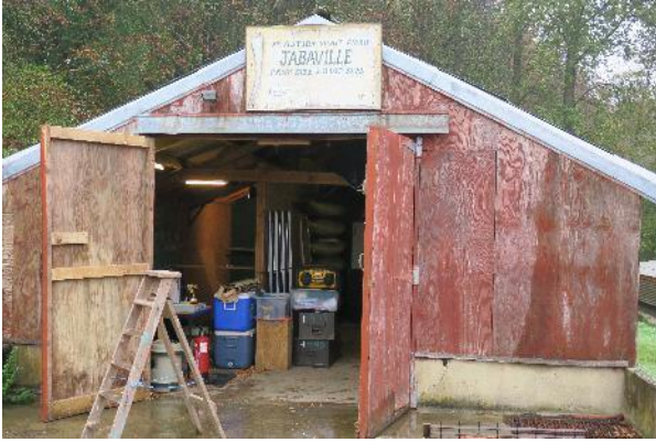
Photograph 1. Building A viewed from the south.
