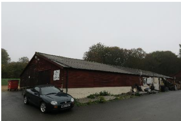
Photograph 11. Building G viewed from the south-east.
