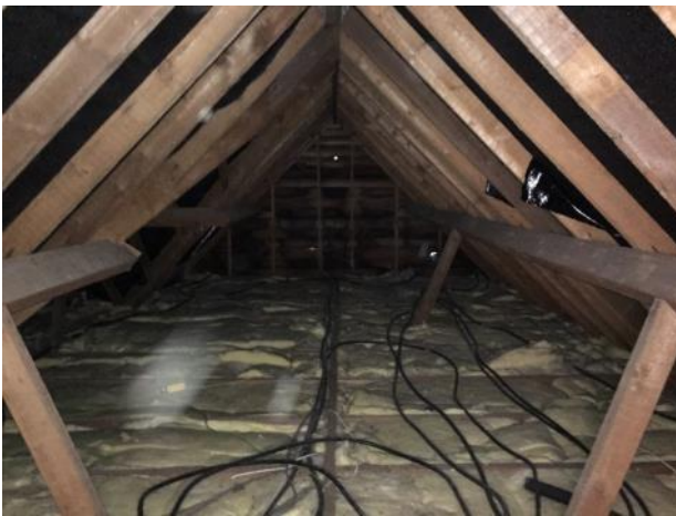
Photograph 3. Loft void within Building F
