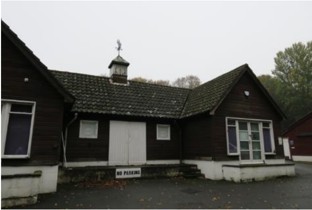
Photograph 1. Building F viewed from the east
