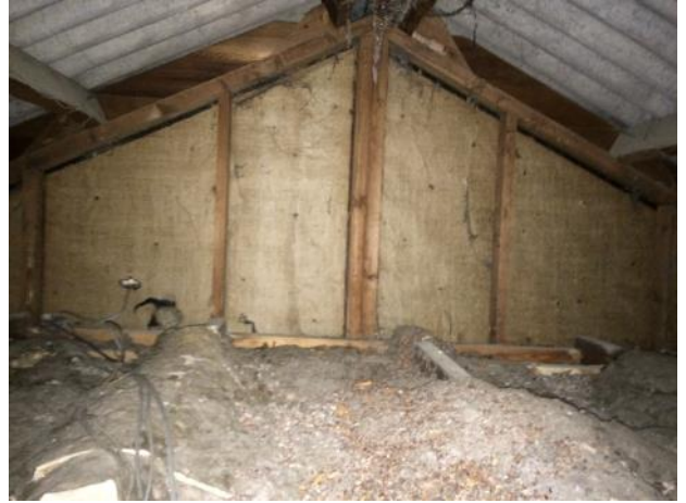
Photograph 8. The loft space within the northern section of Building D.
