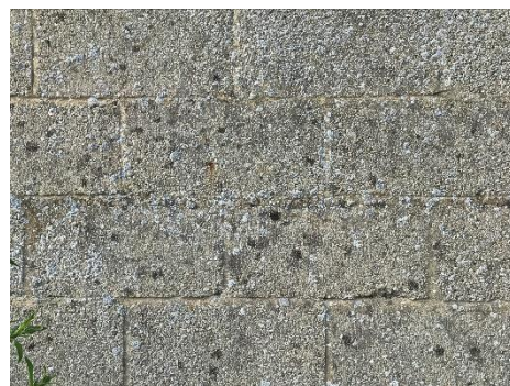
Typical existing concrete block detail (before repointing)
