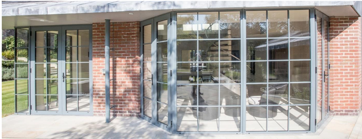
Typical detail of Crittal-type windows (to illustrate style, colour to be RAL7016, Anthracite, see below)
