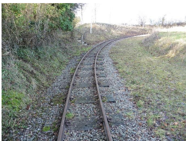
Photo 5: Railway line with edges of ephemeral vegetation.
