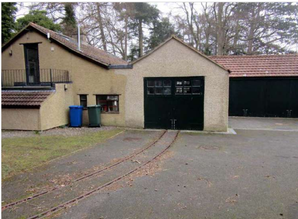
Image 2: Outbuildings northeast of the house.
