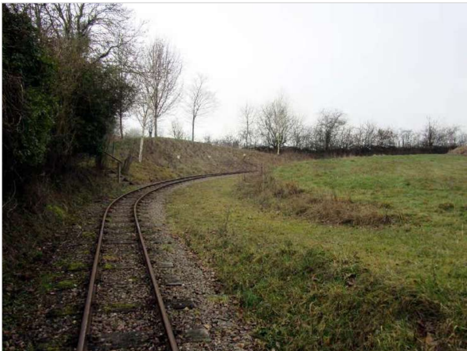
Image 8: Looking west up the incline towards the southwest angle of the site.
