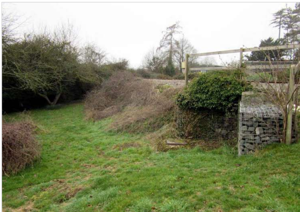
Image 4: The railway track running on an embankment around the southeast side of the garden.
