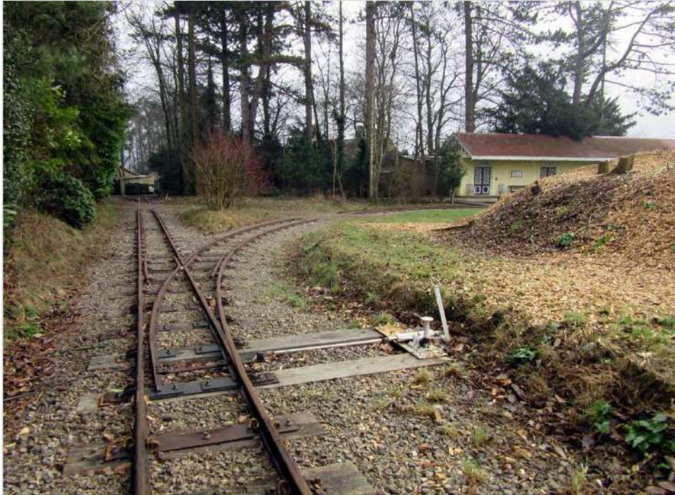
Image 11: Looking east-southeast down to the outbuildings (left) and the curve / crossing to the station (right).
