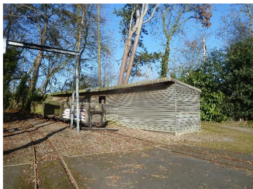
Photo 21: Building 7, southern elevation
