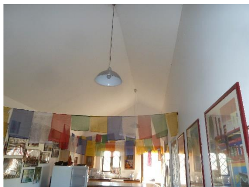
Photo 5: Building 2 internal, plastered ceiling
