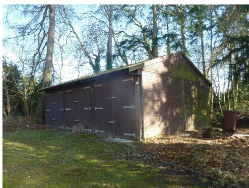
Photo 19: Building 6 west and south elevations
