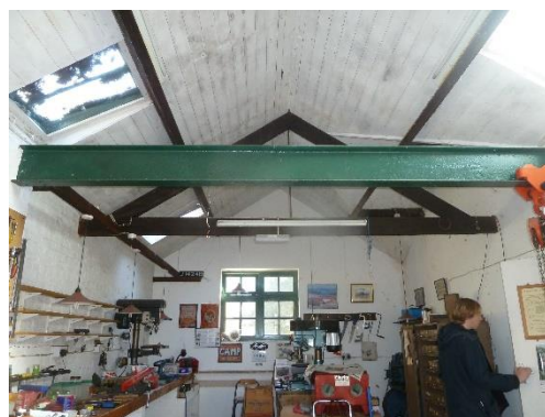
Photo 17: Building 5 interior - workshop
